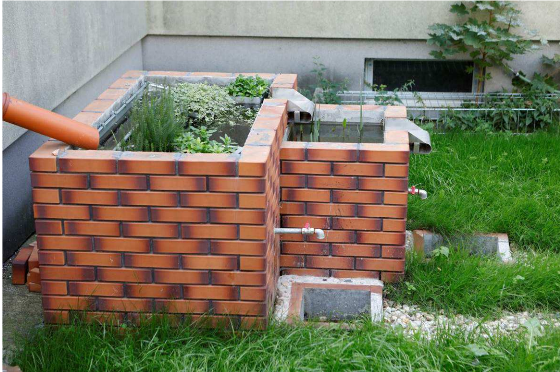
Photo 7 State of the site after the works - Climabox
