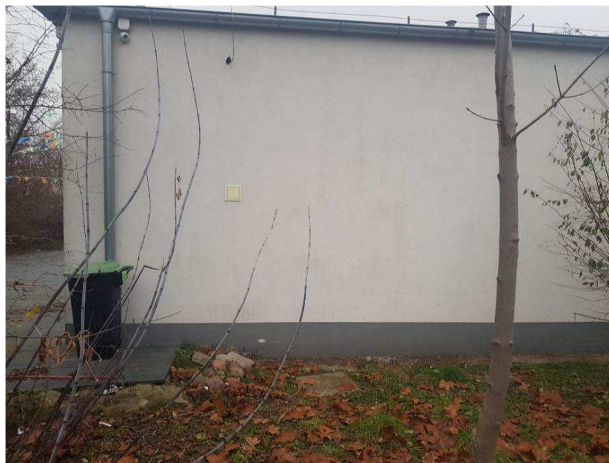
Photo 2 State of the site before execution of the works
