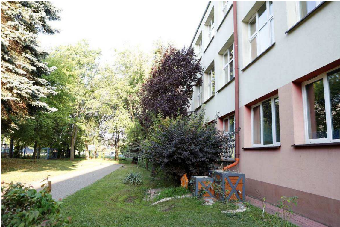
Photo 4 State of the site after the works - Climabox + swale
