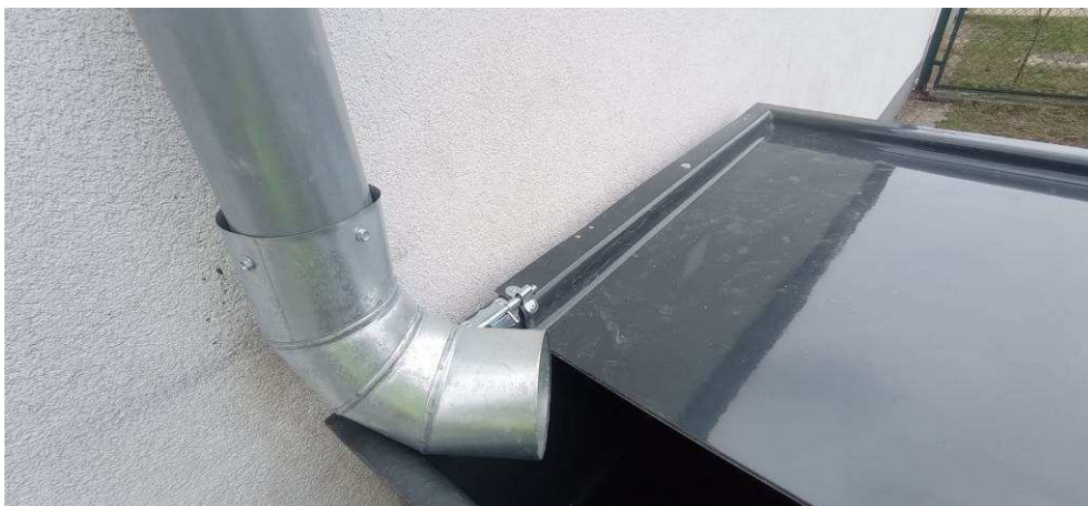
Photo 11 State of the site after the works - drain connection
