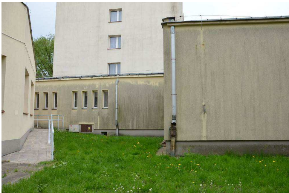
Photo 2 State of the site before the works - Climabox
