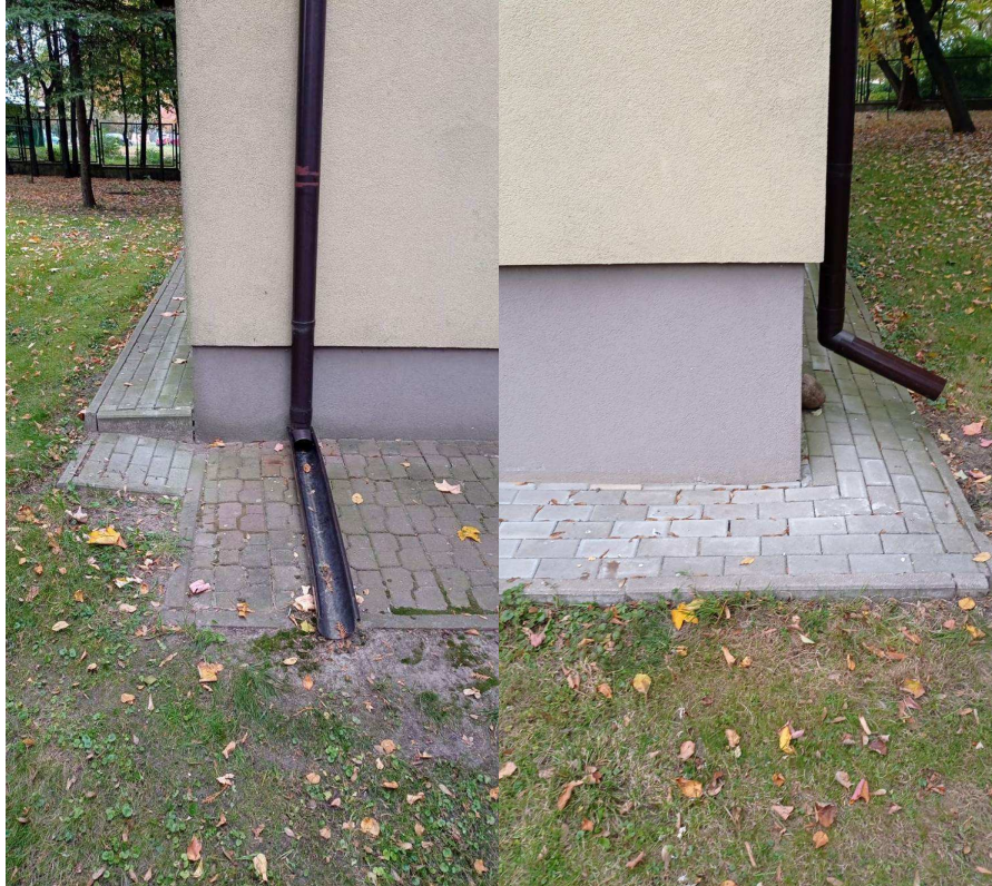
Photo 1, 2 State of the site before the works - Climabox
