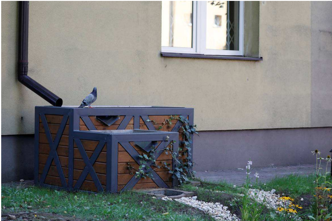
Photo 25 State of the site after the works – Climabox and swale
