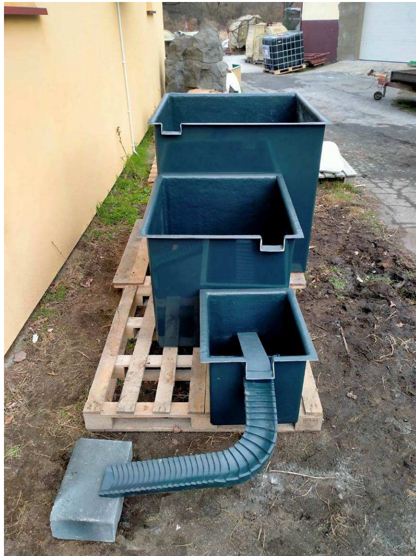
Photo 7 State of the site during the execution of works - Preparation of the Climabox; in the foreground the amphibian ladder
