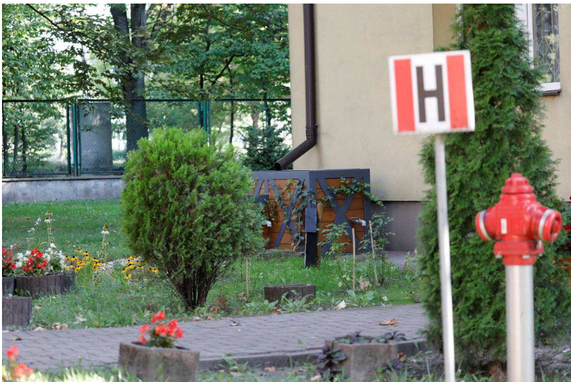
Photo 24 State of the site after the works – Climabox and swale
