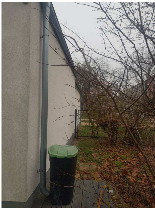
Photo State of the site before execution of the works
