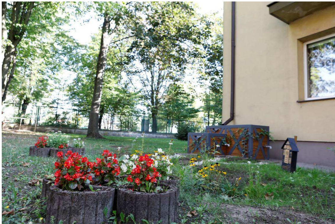
Photo 28 State of the site after the works – Climabox and swale
