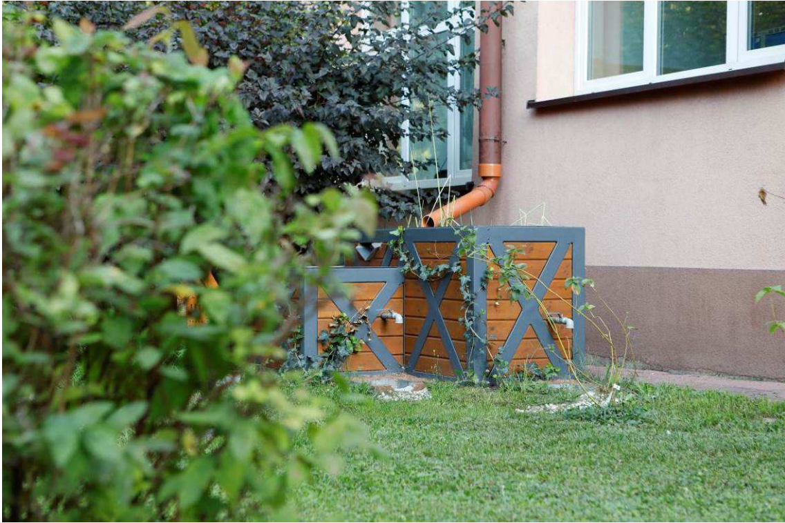
Photo 3 State of the site after the works - Climabox + swale
