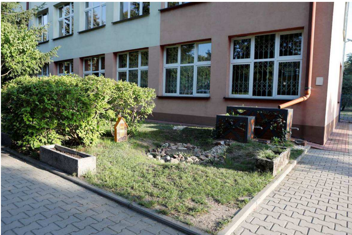
Photo 6 State of the site after the works - Climabox + swale
