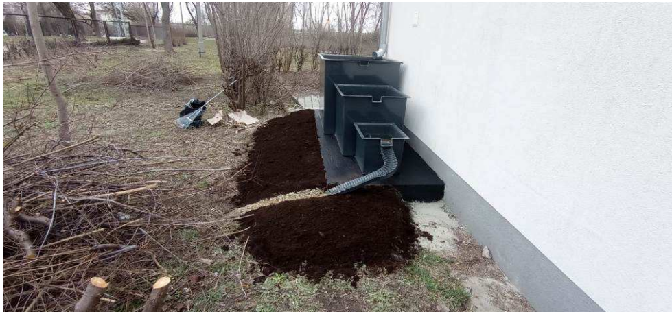
Photo 9 State of the site after the works - general view
