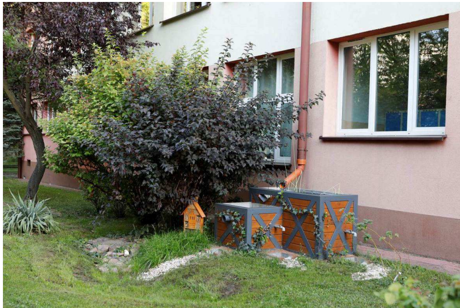
Photo 1 State of the site after the works - Climabox + swale
