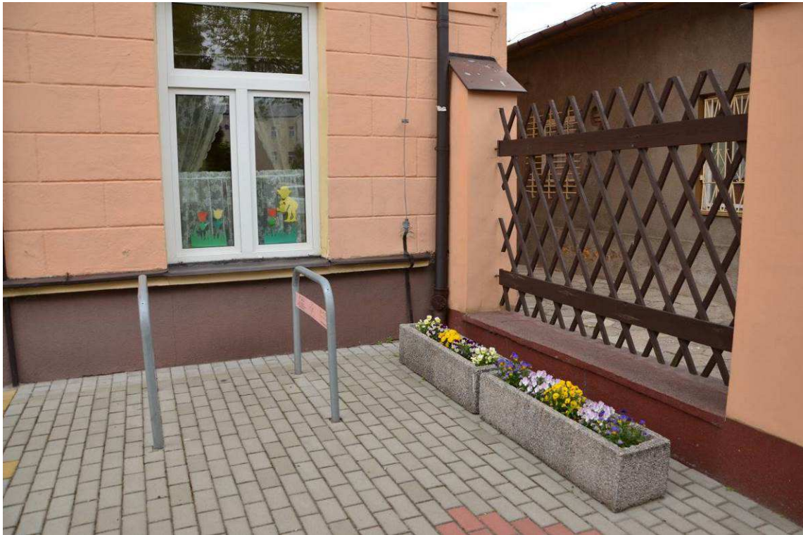
Photo 3 State of the site before execution of the works - Climabox
