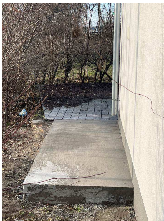
Photo 4 State of the ground during the execution of works - Concrete foundation
