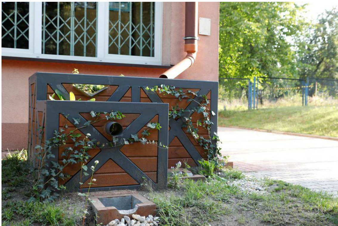
Photo 10 State of the site after the works - Climabox + swale
