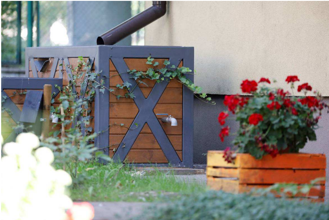
Photo 23 State of the site after the works – Climabox and swale
