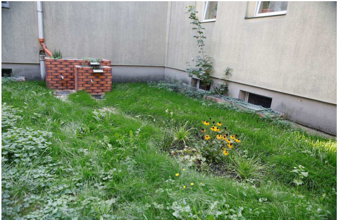
Photo 5 State of the site after the works – Climabox + swale
