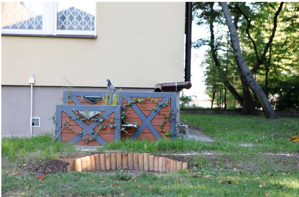
Photo 8 State of the site after the works - Climabox + swale
