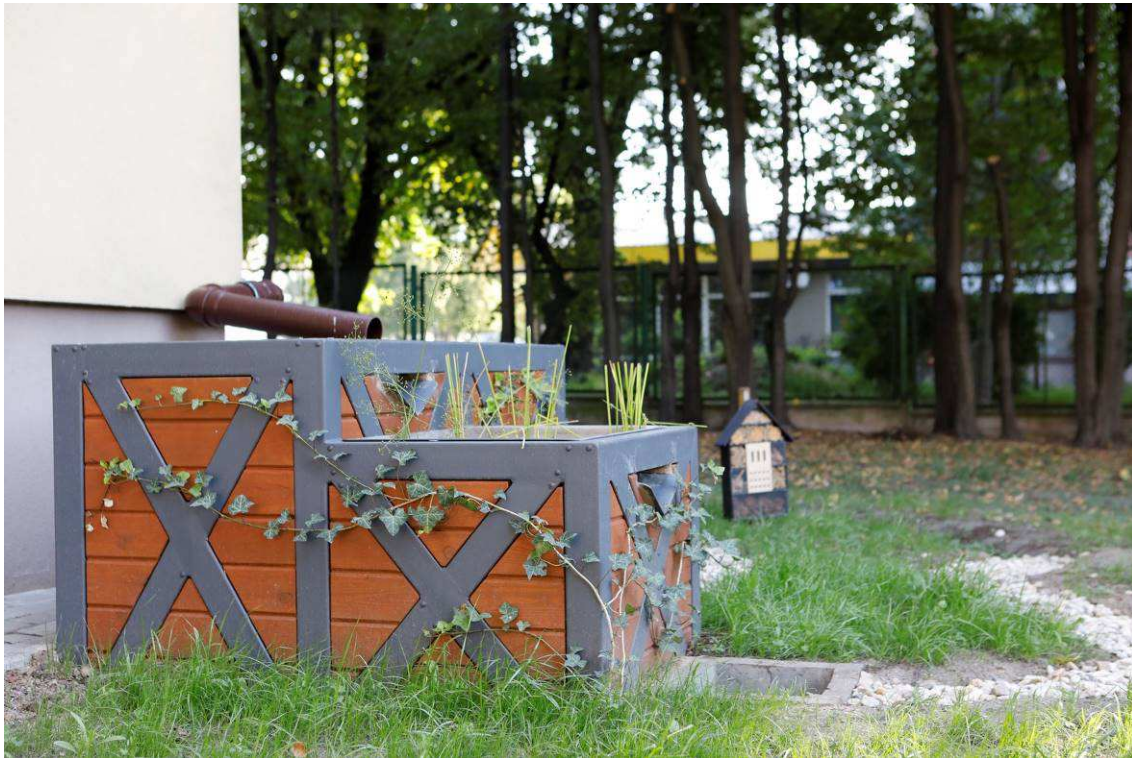
Photo 13 State of the site after the works - Climabox + swale + insect house
