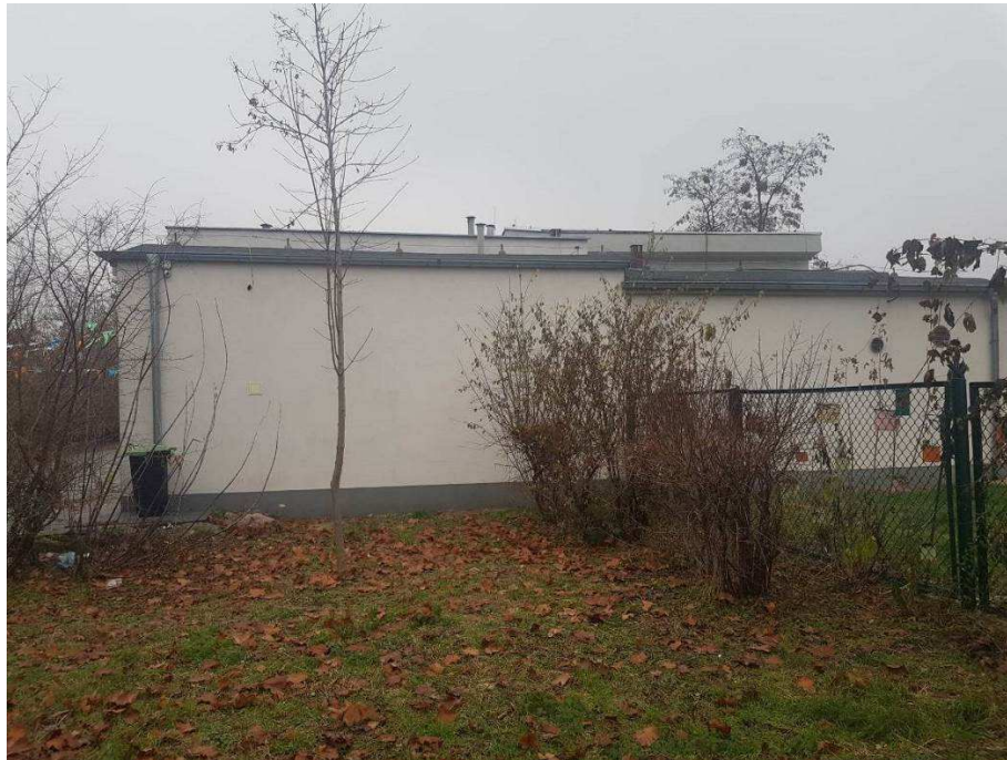
Photo 1 State of the site before execution of the works
