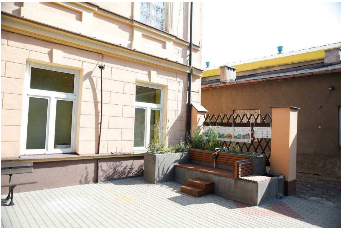
Photo 6 State of the site after the works - Climabox + bench
