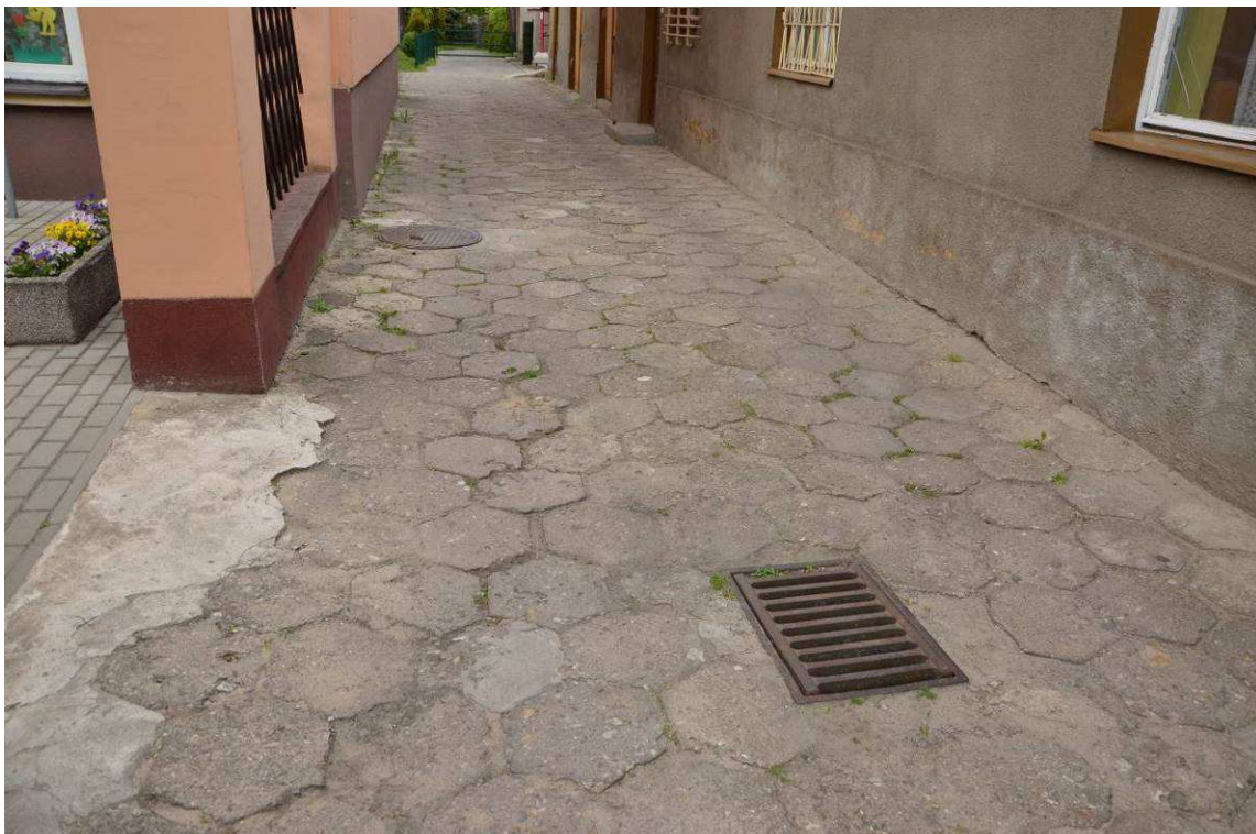
Photo 4 State of the site before execution of the works - Climabox
