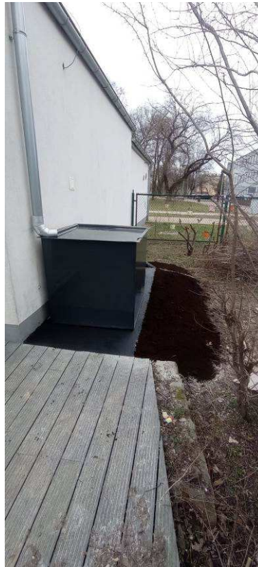
Photo 12 State of the site after the works – general view
