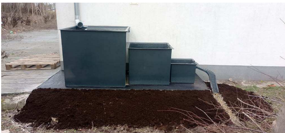
Photo 8 State of the site after the works - general view
