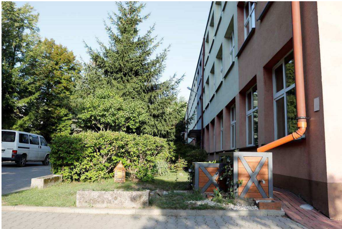
Photo 7 State of the site after the works - Climabox + swale
