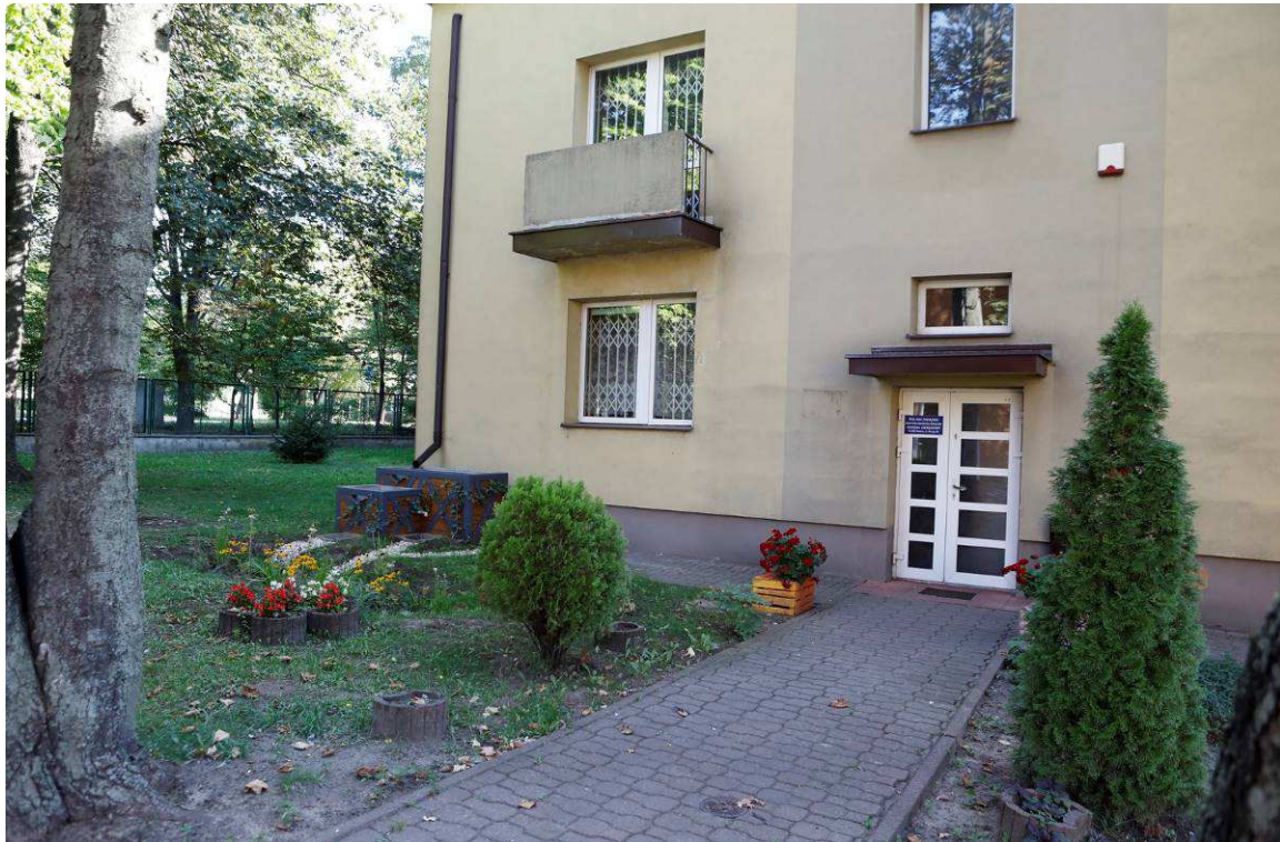
Photo 27 State of the site after the works – Climabox and swale
