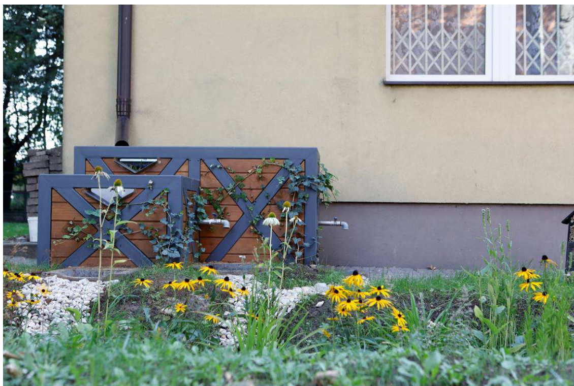
Photo 29 State of the site after the works – Climabox and swale
