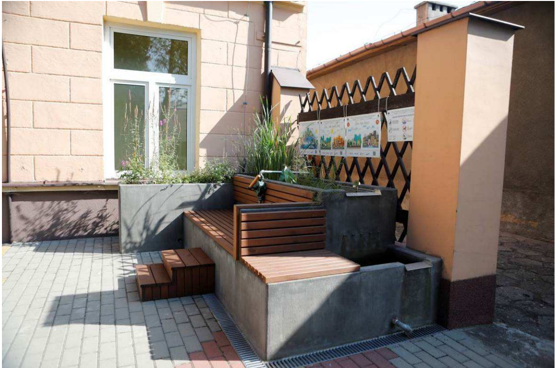
Photo 5 State of the site after the works - Climabox + bench
