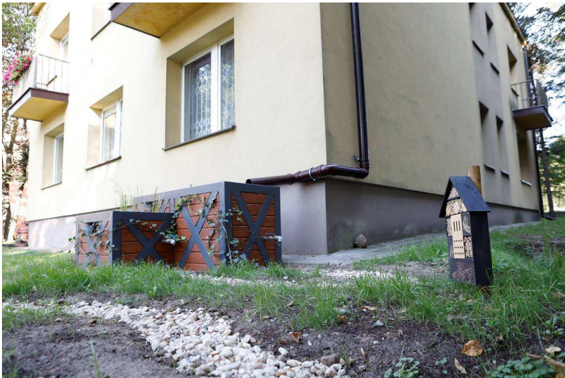
Photo 10 State of the site after the works - Climabox + swale + insect house
