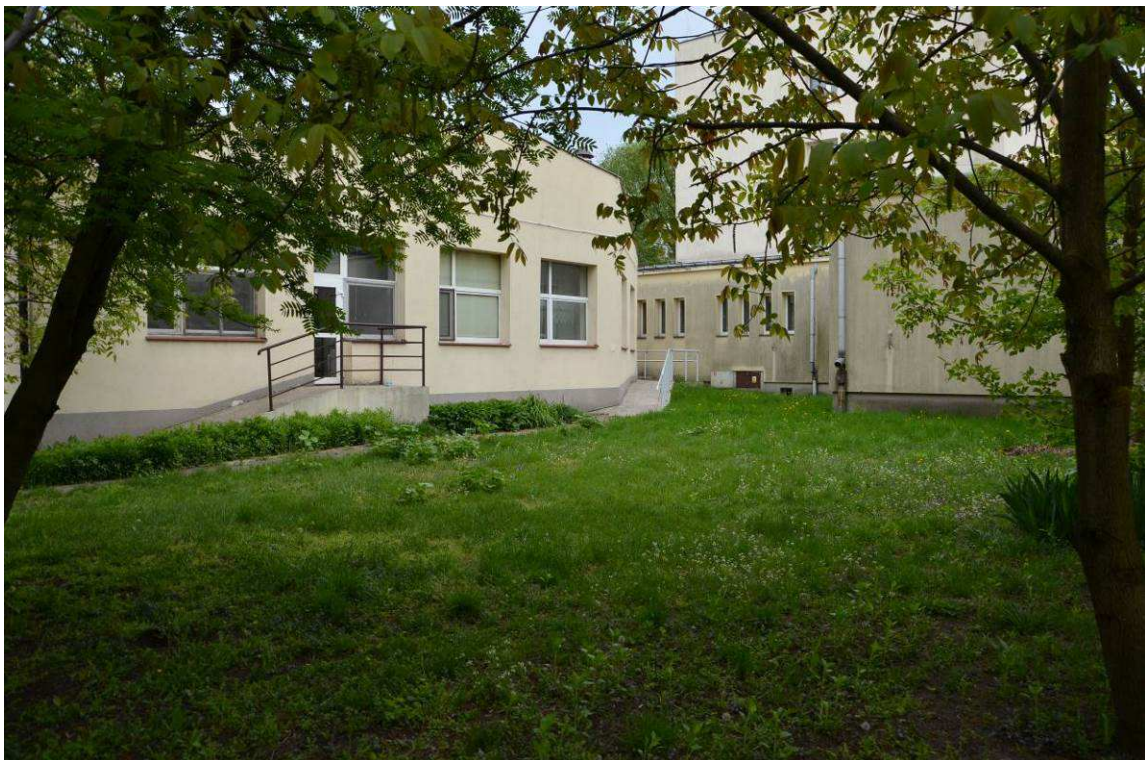
Photo 4 State of the site before the works - Climabox
