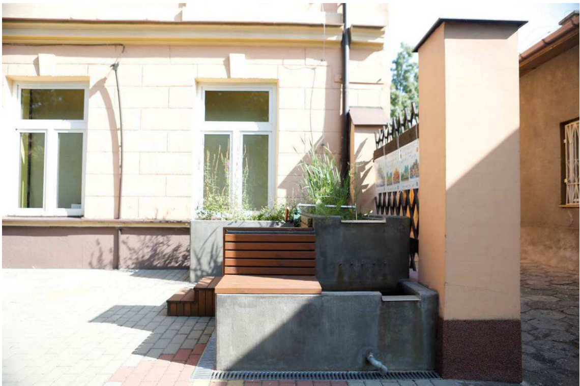
Photo 8 State of the site after the works - Climabox + bench
