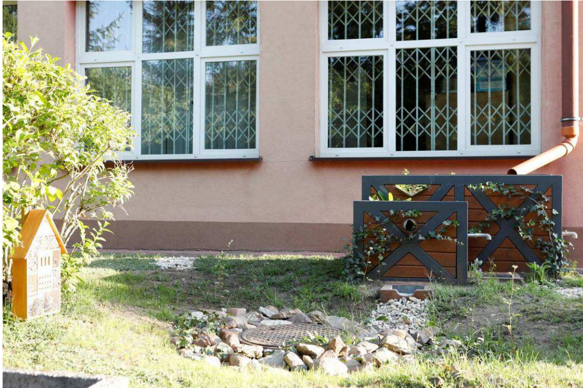
Photo 9 State of the site after the works - Climabox + swale
