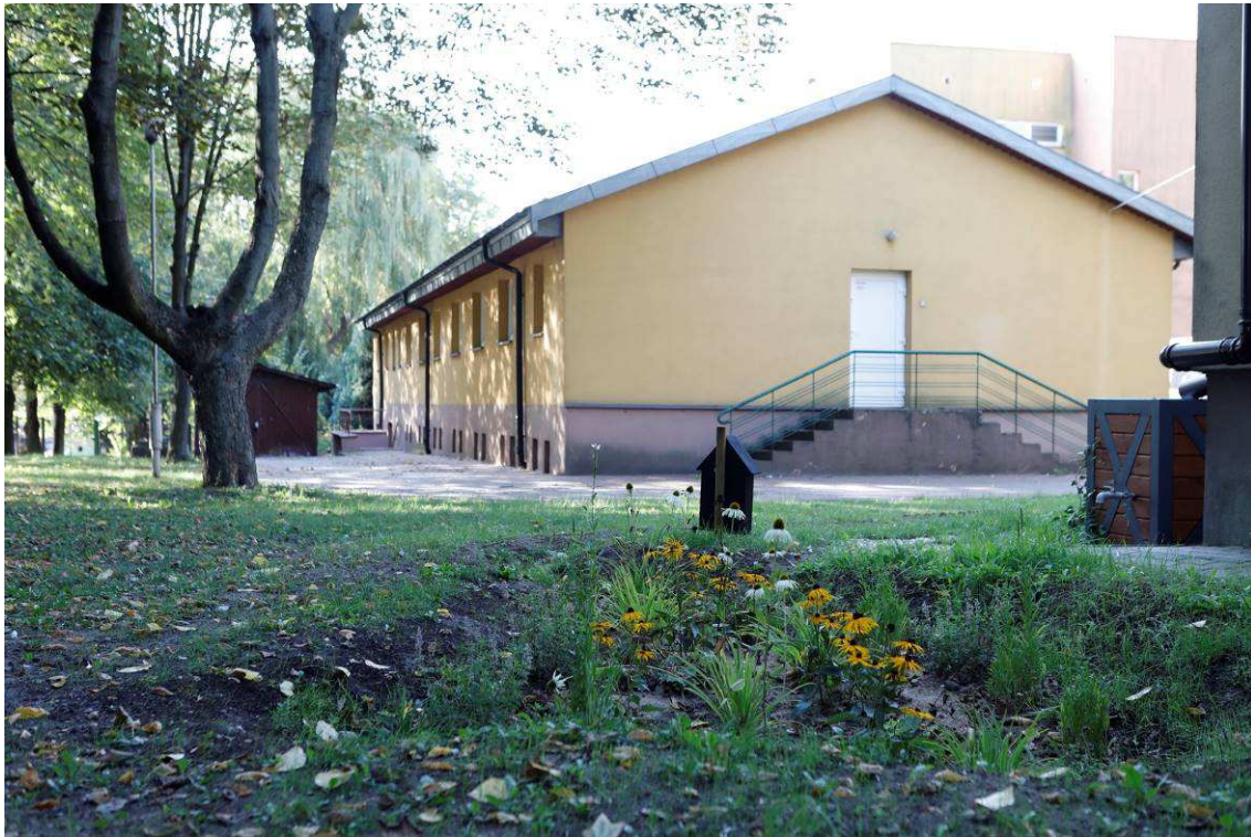
Photo 11 State of the site after the works - biodiversity effect
