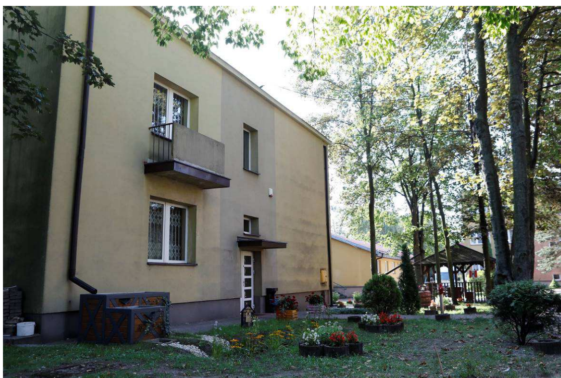
Photo 30 State of the site after the works – Climabox and swale
