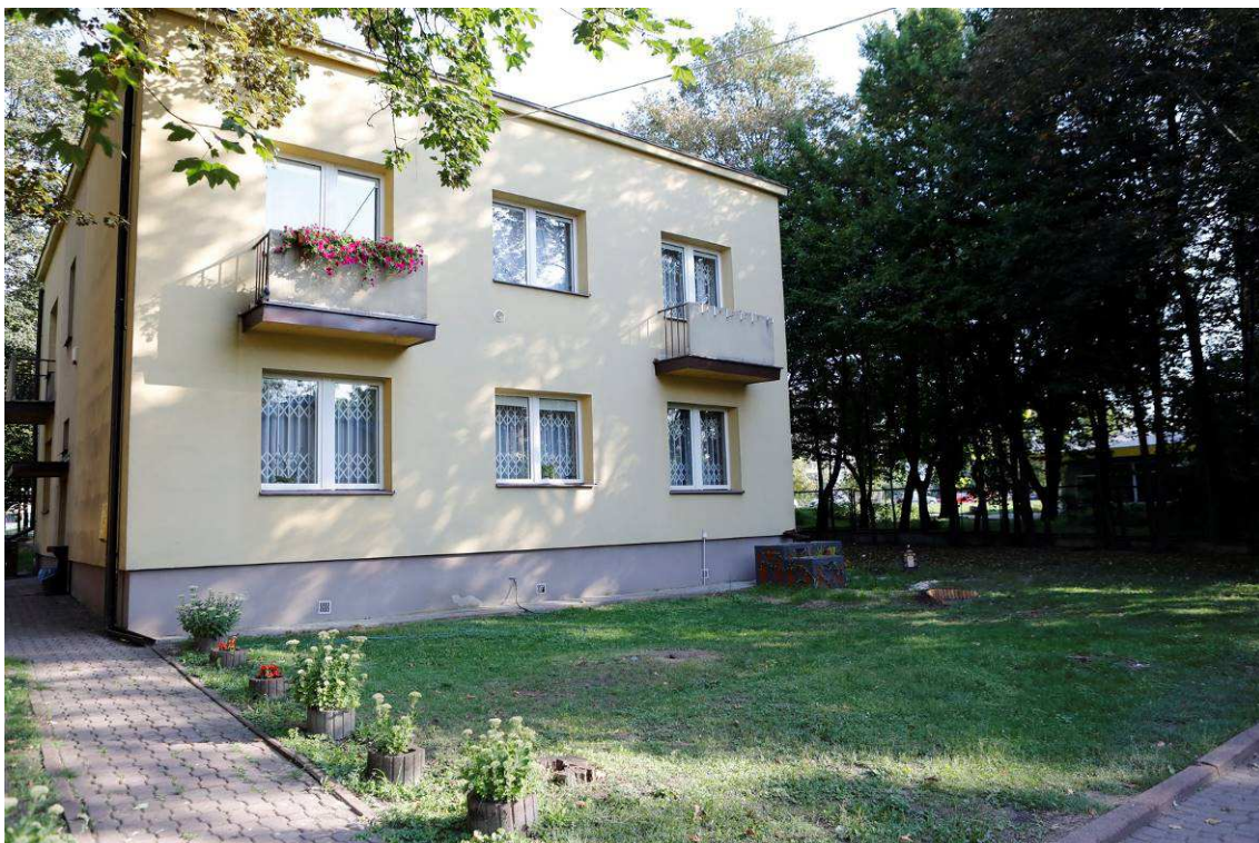
Photo 14 State of the site after the works - Climabox
