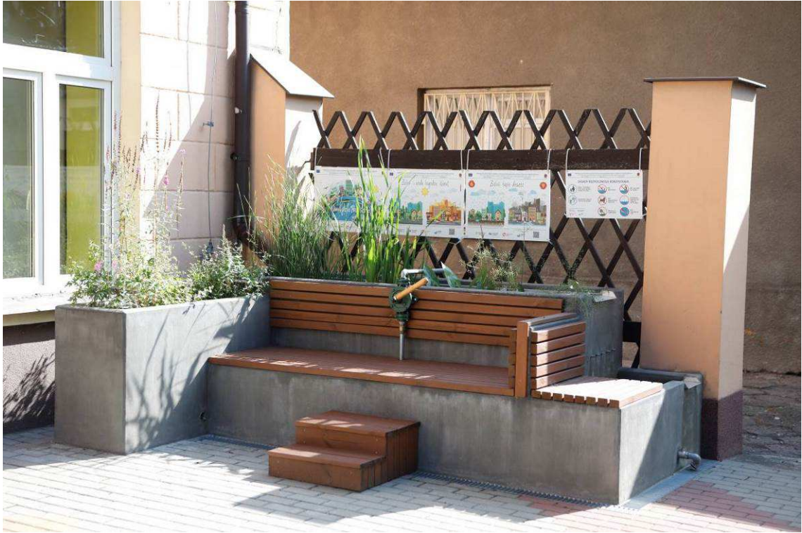
Photo 9 State of the site after the works - Climabox + bench + information boards
