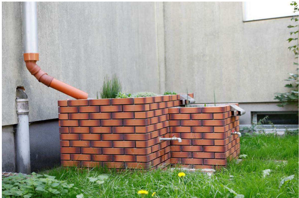
Photo 6 State of the site after the works - Climabox
