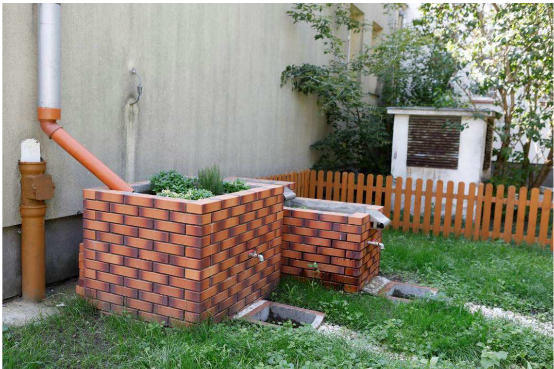
Photo 12 State of the site after the works - Climabox + swale
