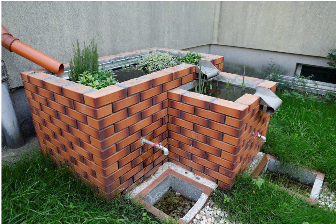
Photo 1 State of the site after the works - Climabox
