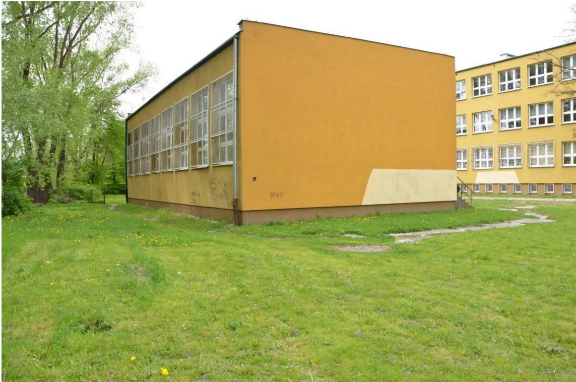
Photo 1 Appearance of the site before construction - Climapond with bench
