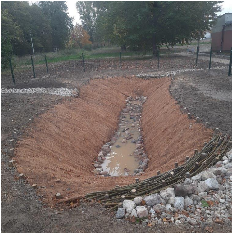
Photo 9 Appearance of the site after construction – Climapond - a dispersing element in the form of a stone dam with a fascine support
