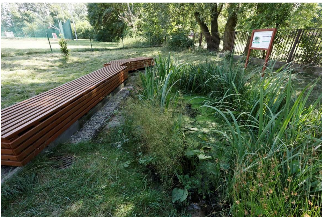
Photo 16 Appearance of the site after the construction - Climapond with bench
