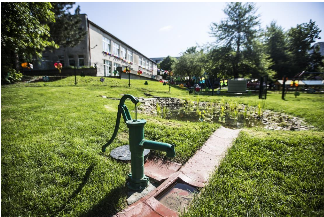
Photo 6 Appearance of the site after the works - Climapond
