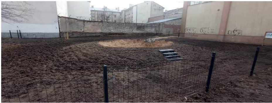
Photo 6 Appearance of the site after completion of the works -Climapond
