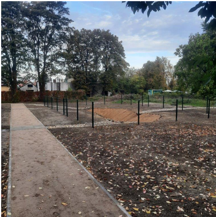
Figure 11 Appearance of the site after construction – Climapond
