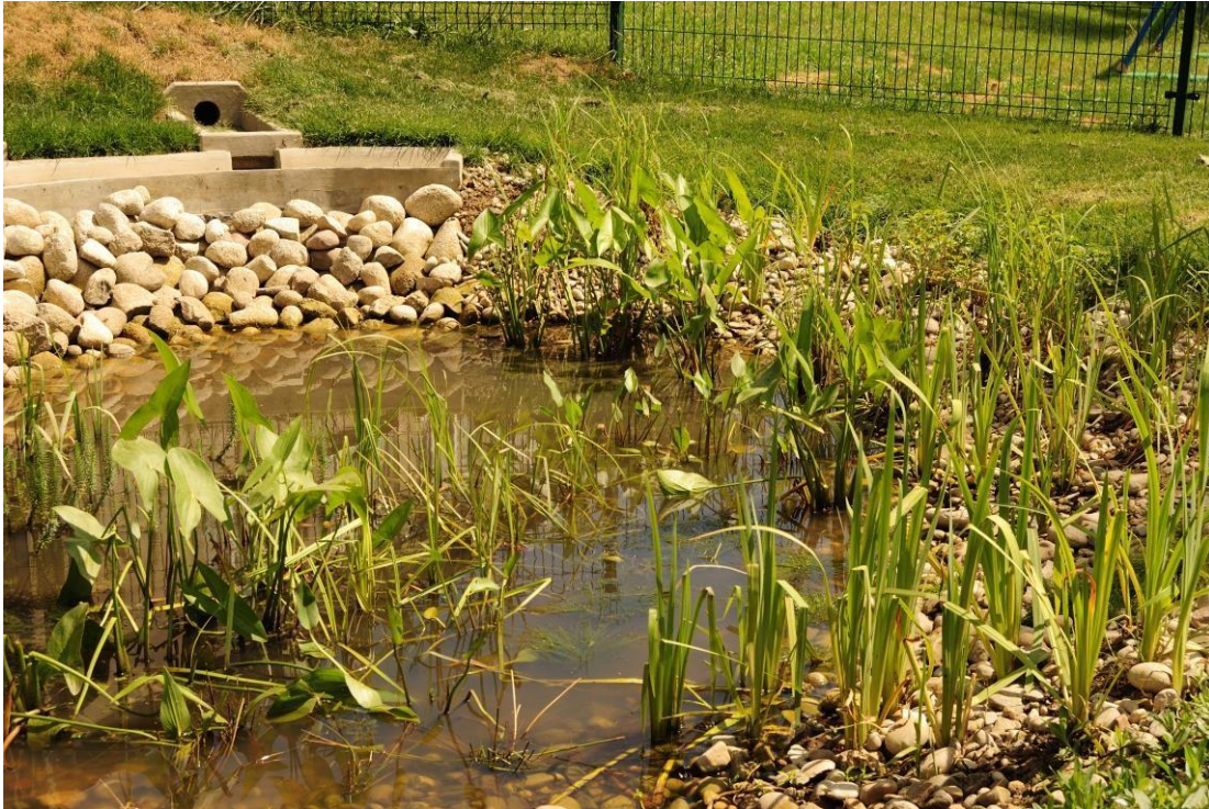
Photo 7 Appearance of the site after the works - Climapond
