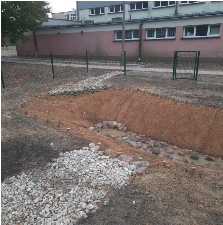
Photo 10 Appearance of the site after construction – Climapond
