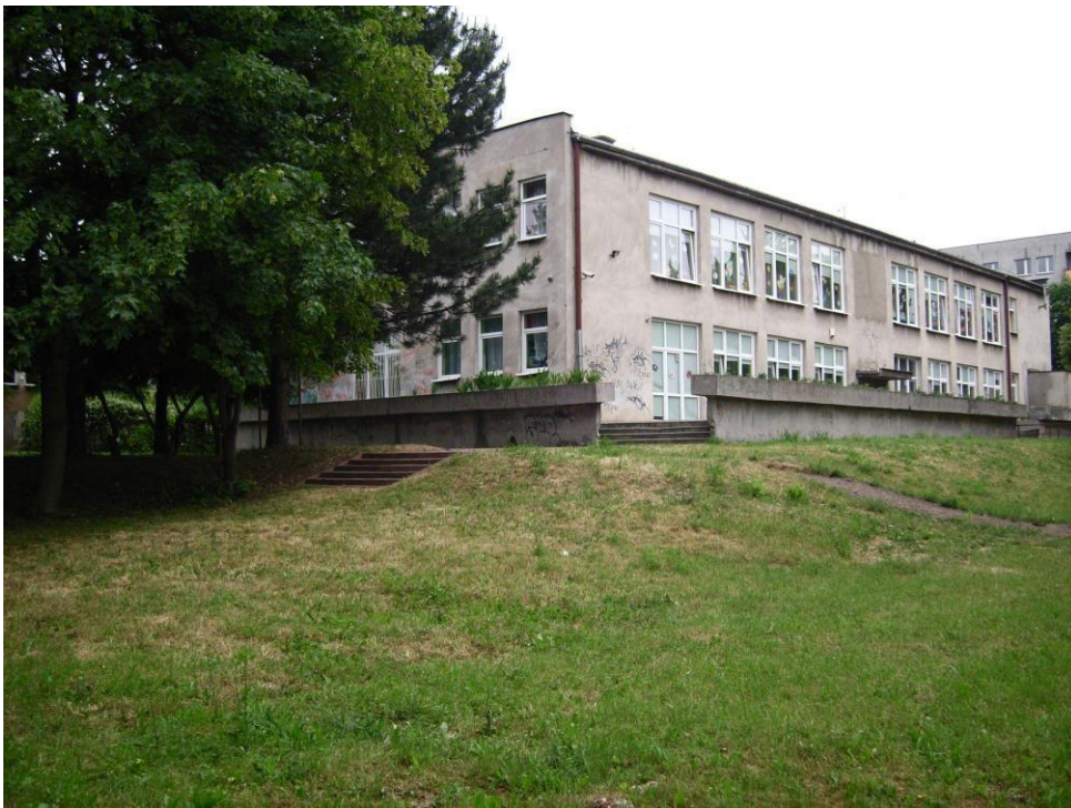
Photo 2 Appearance of the site before construction - Climapond
