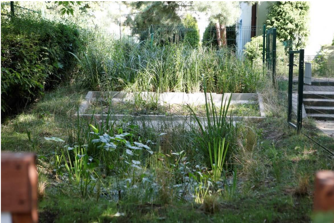
Photo 8 Appearance of the site after the construction – Climapond
