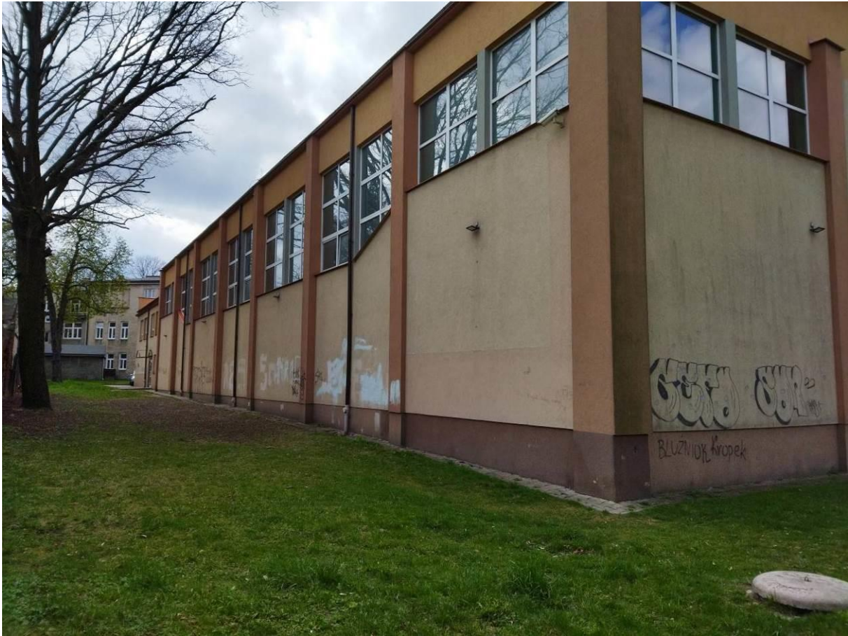
Photo 4 Appearance of the site before construction – Climapond
