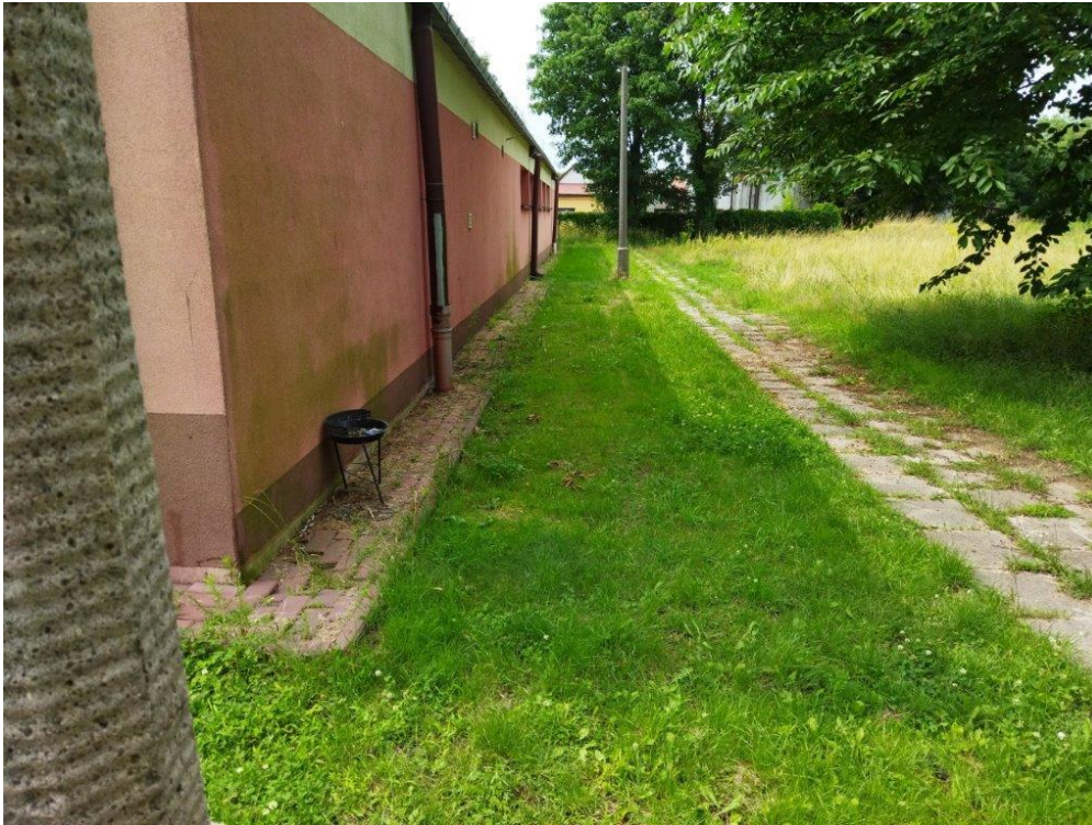
Photo 1 Appearance of the site before construction - Climapond
