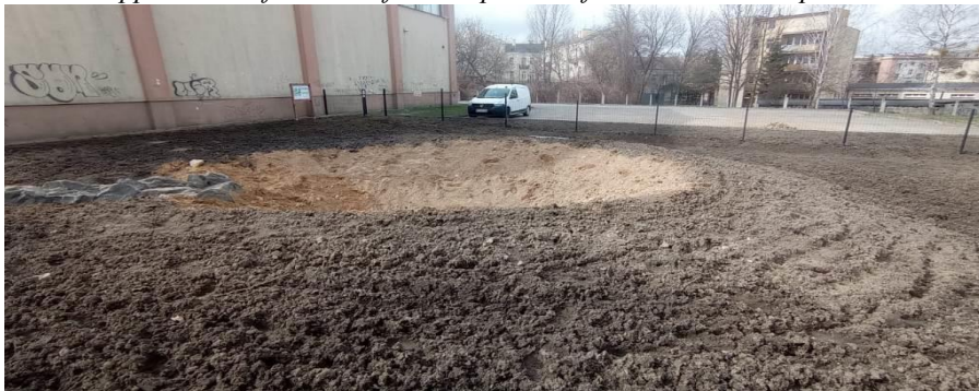
Photo 7 Appearance of the site after completion of the works -Climapond
