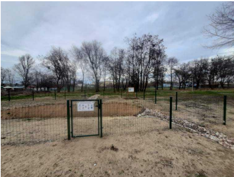
Photo 14 Appearance of the site after construction – safety board at Climapond
