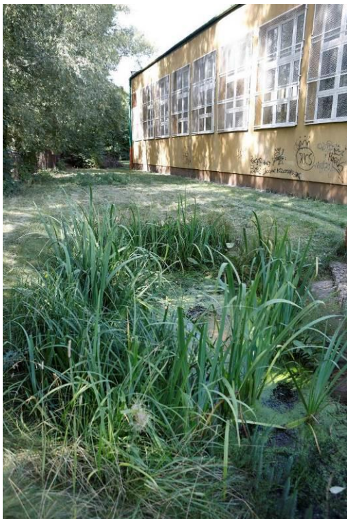
Photo 12 Appearance of the site after the construction - Climapond with bench
