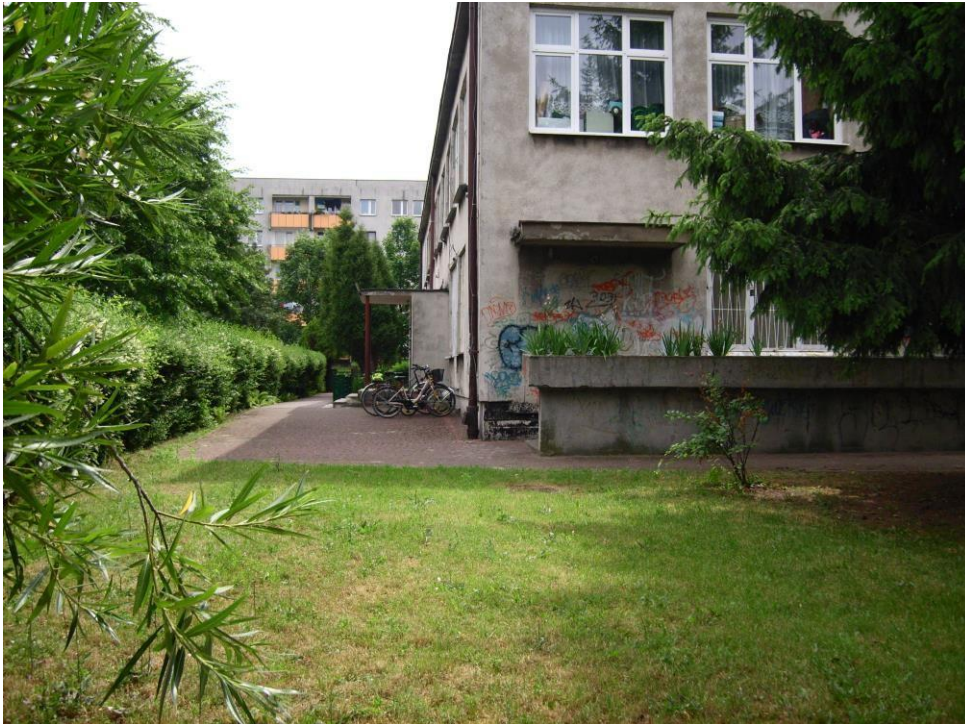
Photo 1 Appearance of the site before construction - Climapond
