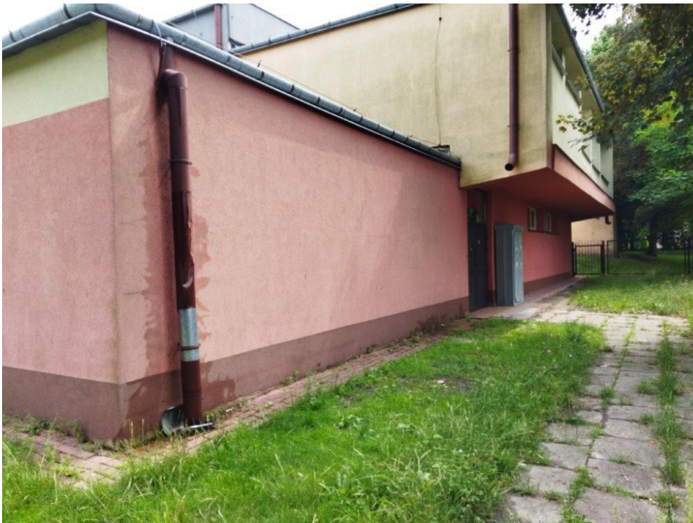
Photo 4 Appearance of the site before construction - Climapond
