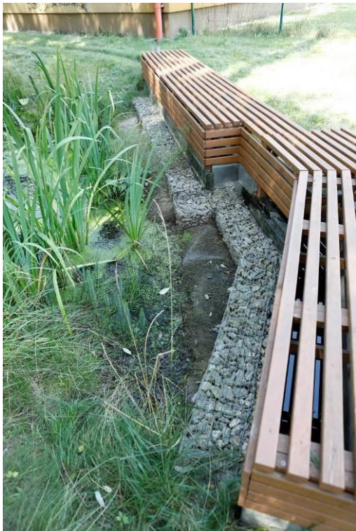
Photo 13 Appearance of the site after the construction - Climapond with bench
