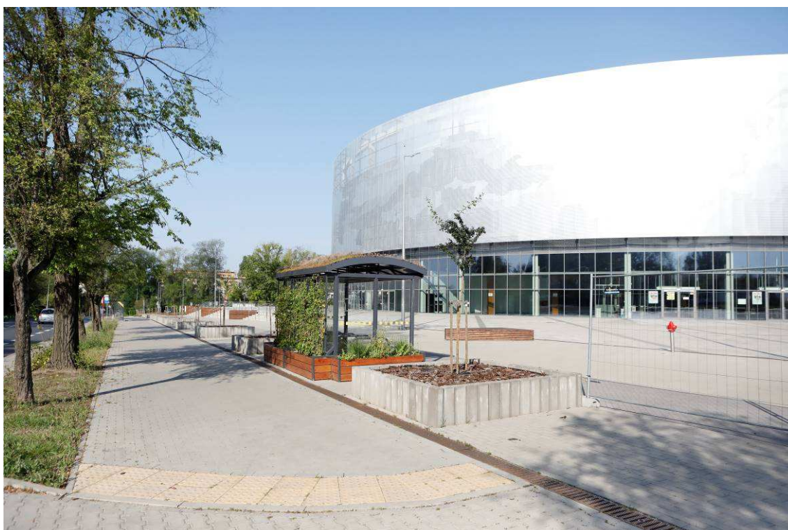
Photo 5 State of the site after the works - Green Bike Shed
