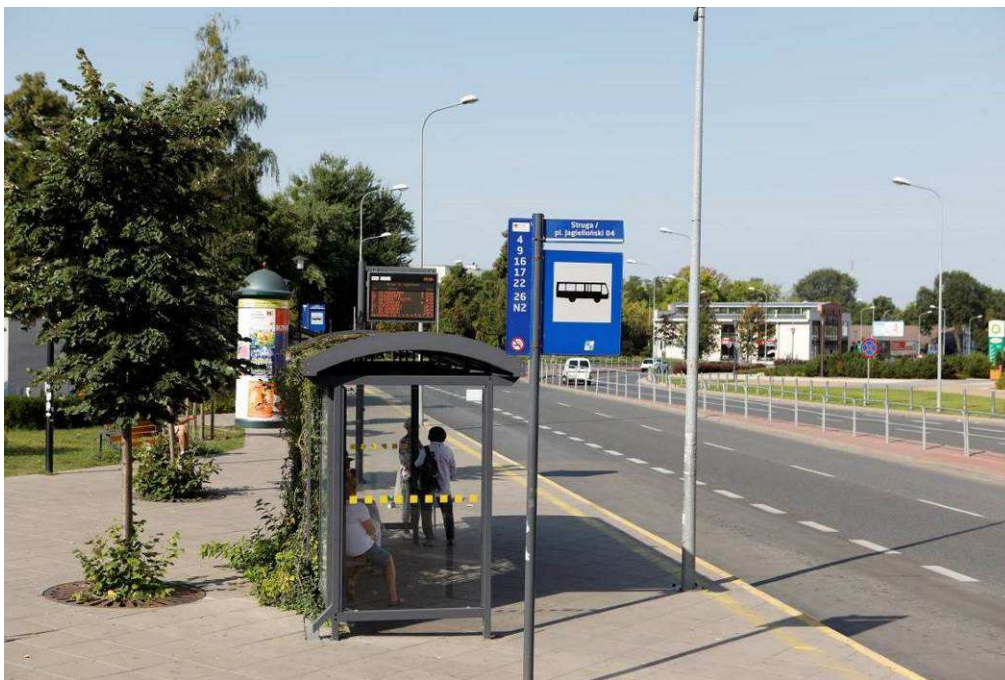
Photo 4 State of the site after the works - Green Bus Shelter with Green Roof and Green Wall
