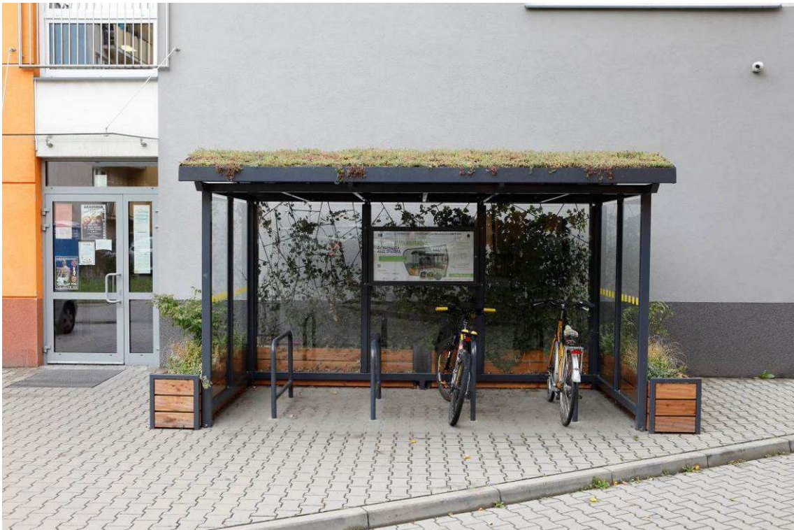
Photo 7 State of the site after completion of works - Green Bike Shelter – Green roof + Planting Pots
