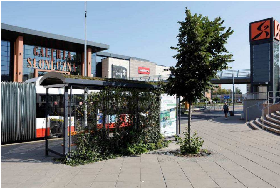
Photo 2 State of the site after the works - Green Bus Shelter with Green Roof and Green Wall
