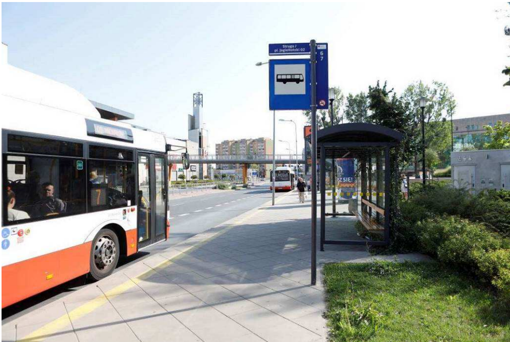
Photo 7 State of the site after the works - Green Bus Shelter with Green Roof and Green Wall
