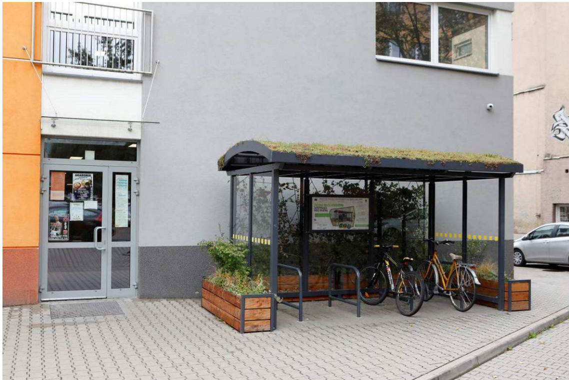
Photo 8 State of the site after completion of works - Green Bike Shelter – Green foot + Planting Pots
