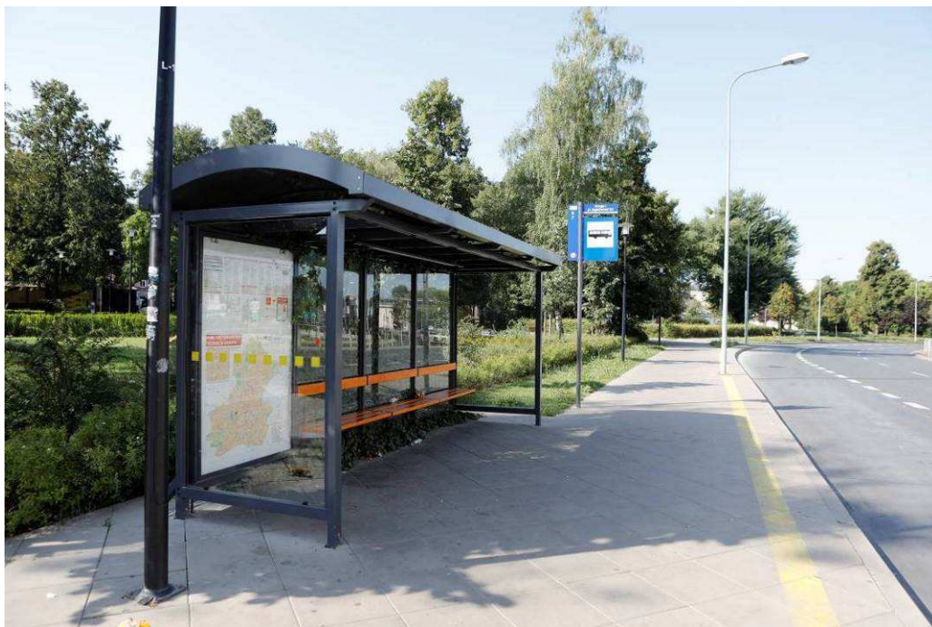
Photo 6 State of the site after the works - Green Bus Shelter with Green Roof and Green Wall
