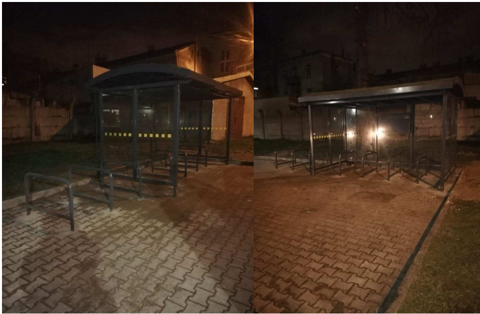
Photos 1, 2 State of the site at the time of the works - Green Bike Shelter
