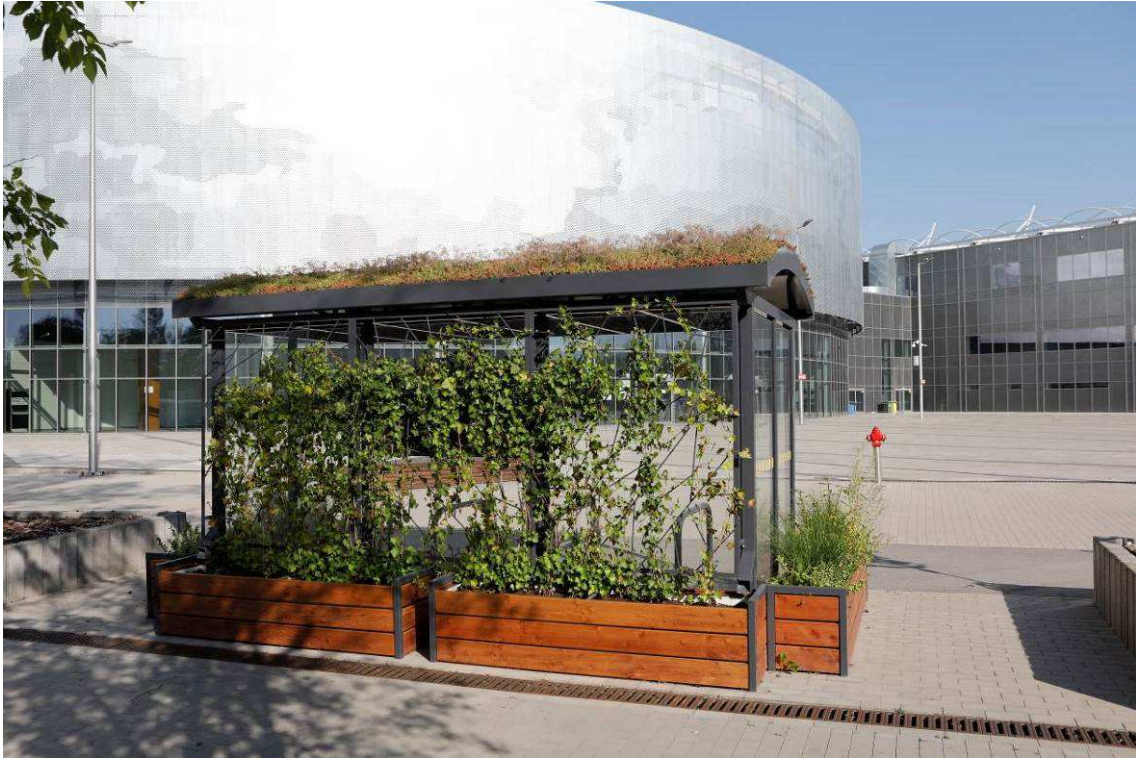
Photo 8 State of the site after the works - Green Bike Shelter - Green Wall + Green Roof
