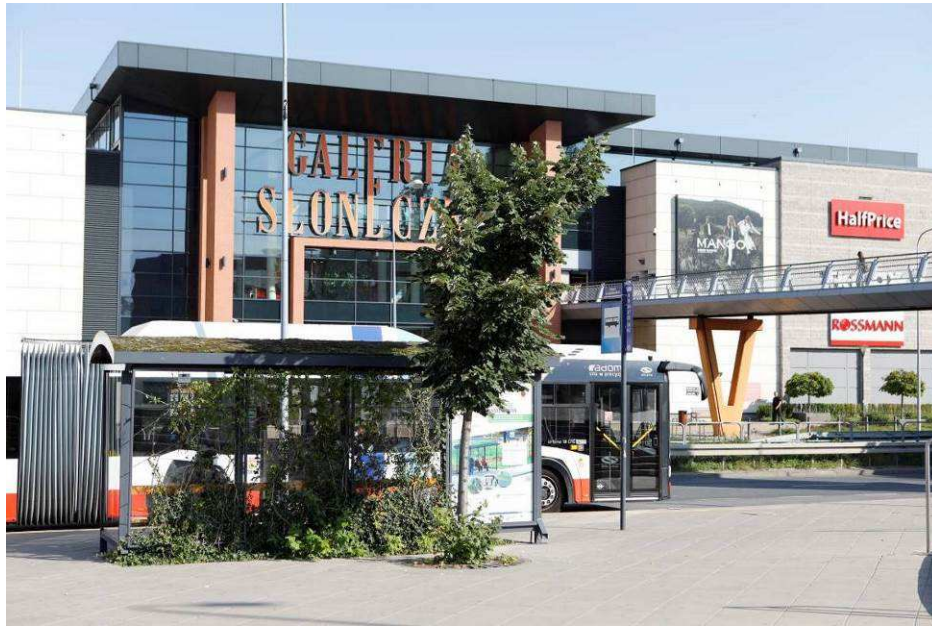
Photo 1 State of the site after the works - Green Bus Shelter with Green Roof and Green Wall
