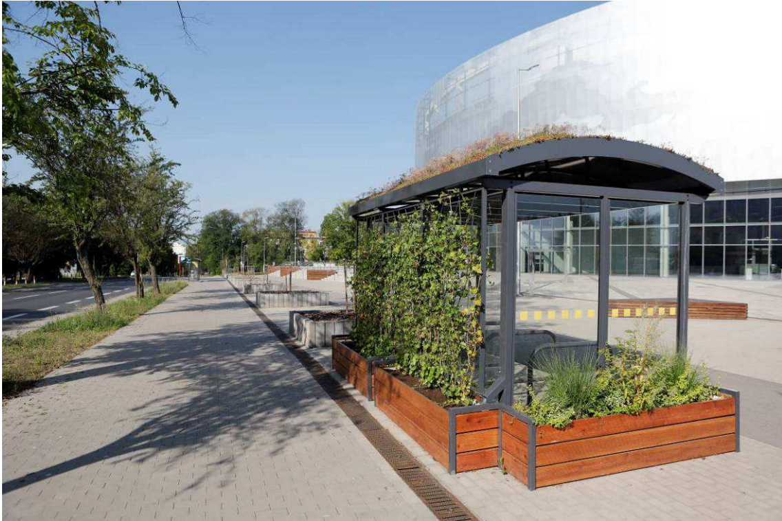
Photo 14 State of the site after the works - Green Bike Shelter – Planting pods +Green Wall
