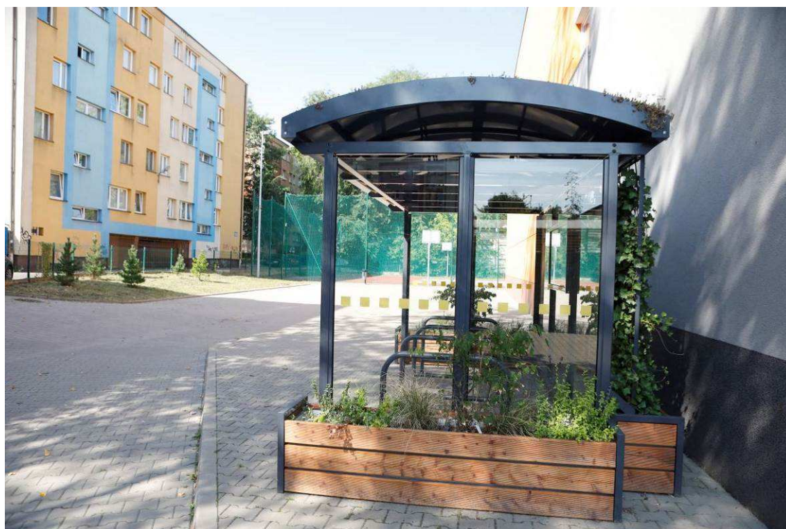
Photo 5 State of the site after the works - Green Bike Shelter – Green wall + Planting Pots
