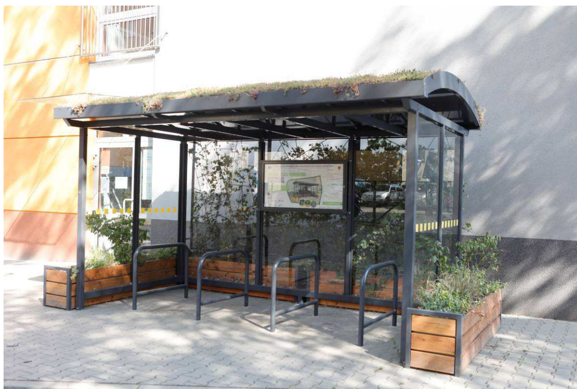
Photo 1 State of the site after the works - Green Bike Shed
