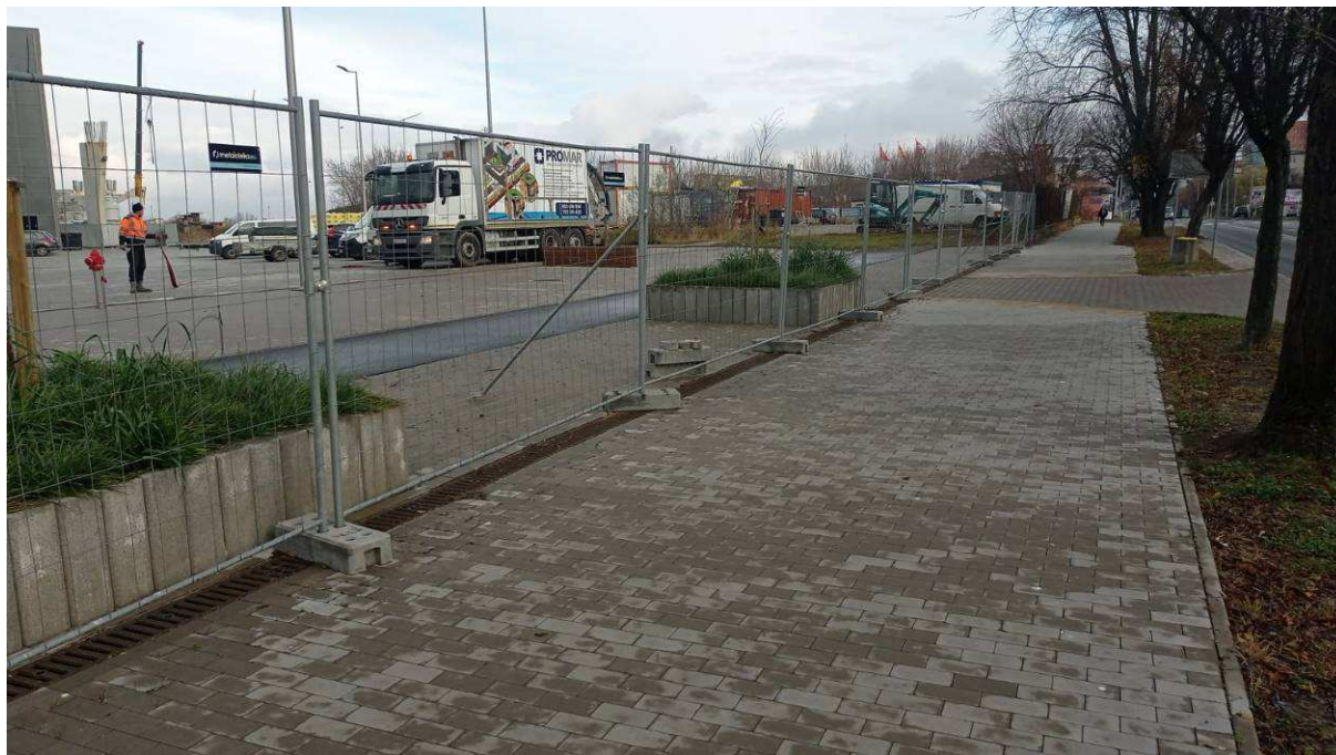
Photo 4 State of the site before works - Green Bike Shed
