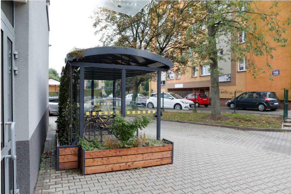
Photo 6 State of the site after the works - Green Bike Shelter – Green wall + Planting Pots
