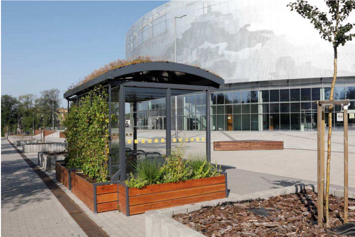
Photo 6 State of the site after the works - Green Bike Shed
