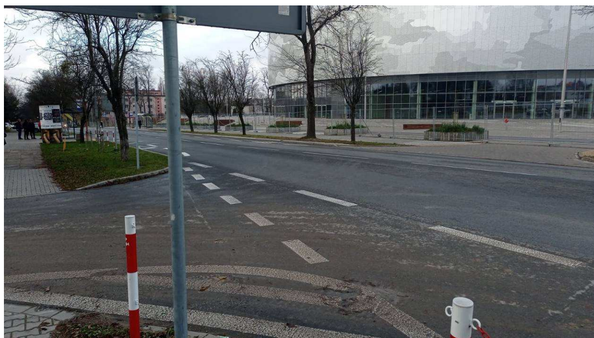
Photo 1 State of the site before works - Green Bike Shed
