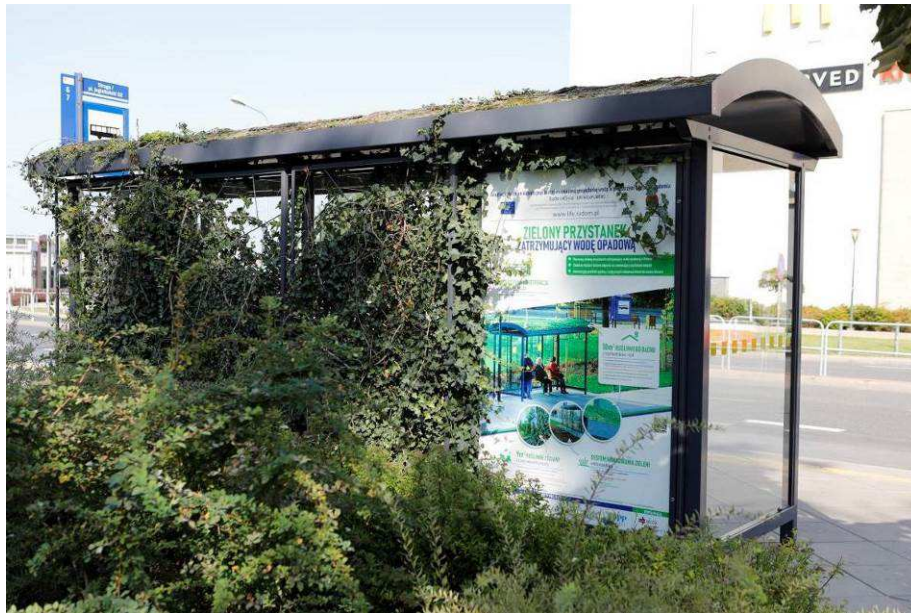
Photo 11 State of the site after the works - Green Bus Shelter with Green Roof and Green Wall - planting of plants
