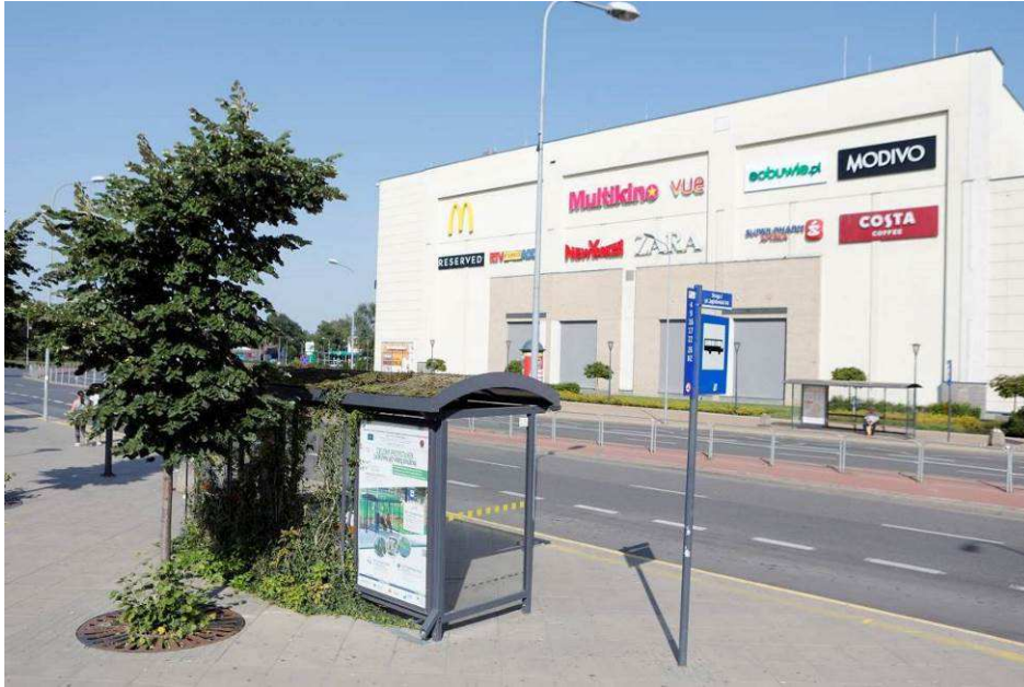
Photo 3 State of the site after the works - Green Bus Shelter with Green Roof and Green Wall
