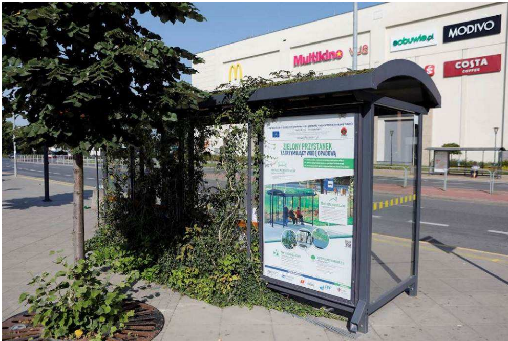
Photo 5 State of the Site after Works - Green Bus Shelter with Green Roof and Green Wall - Information Poster
