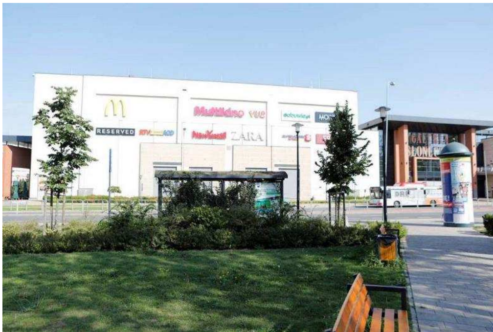
Photo330 Appearance of the site after the construction- Rain garden in the basin behind the shelter
