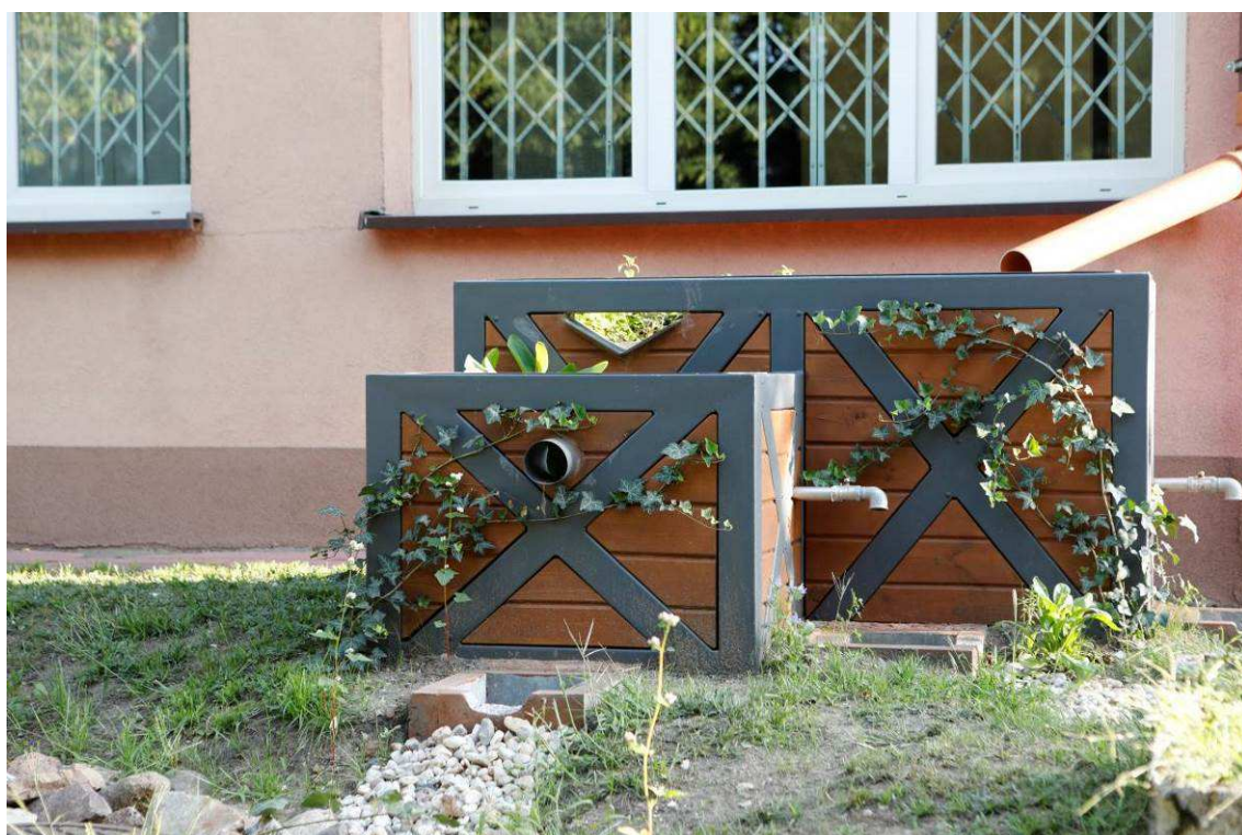
Picture 4 Appearance of the area after the construction- Climabox + Swale
