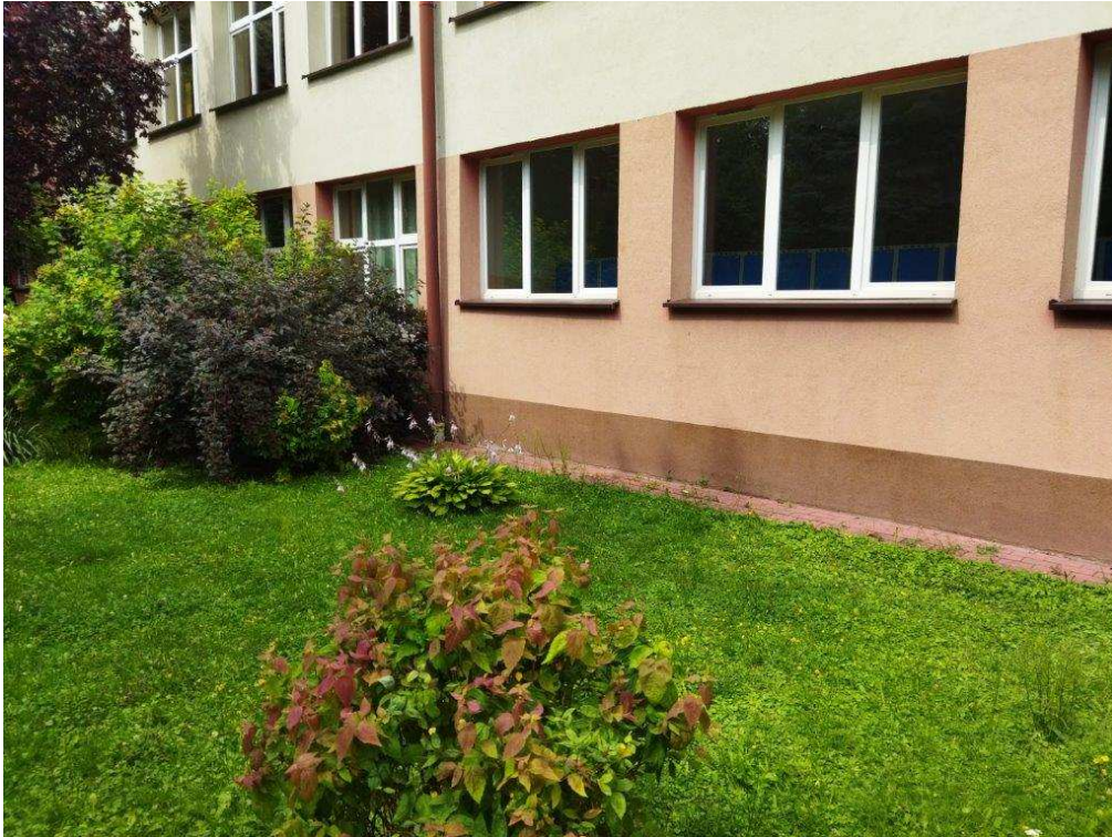
Picture45 area before the construction- Swale
