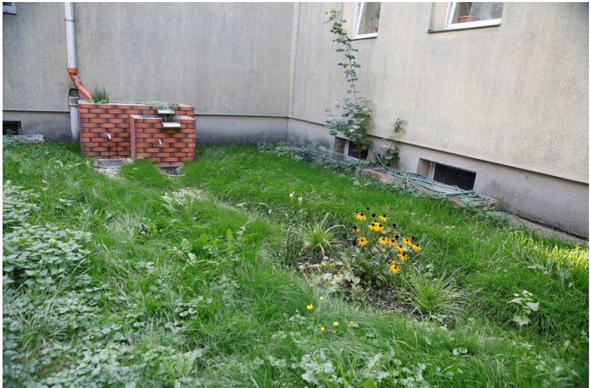
Picture40 Appearance of the area after the construction- Swale
