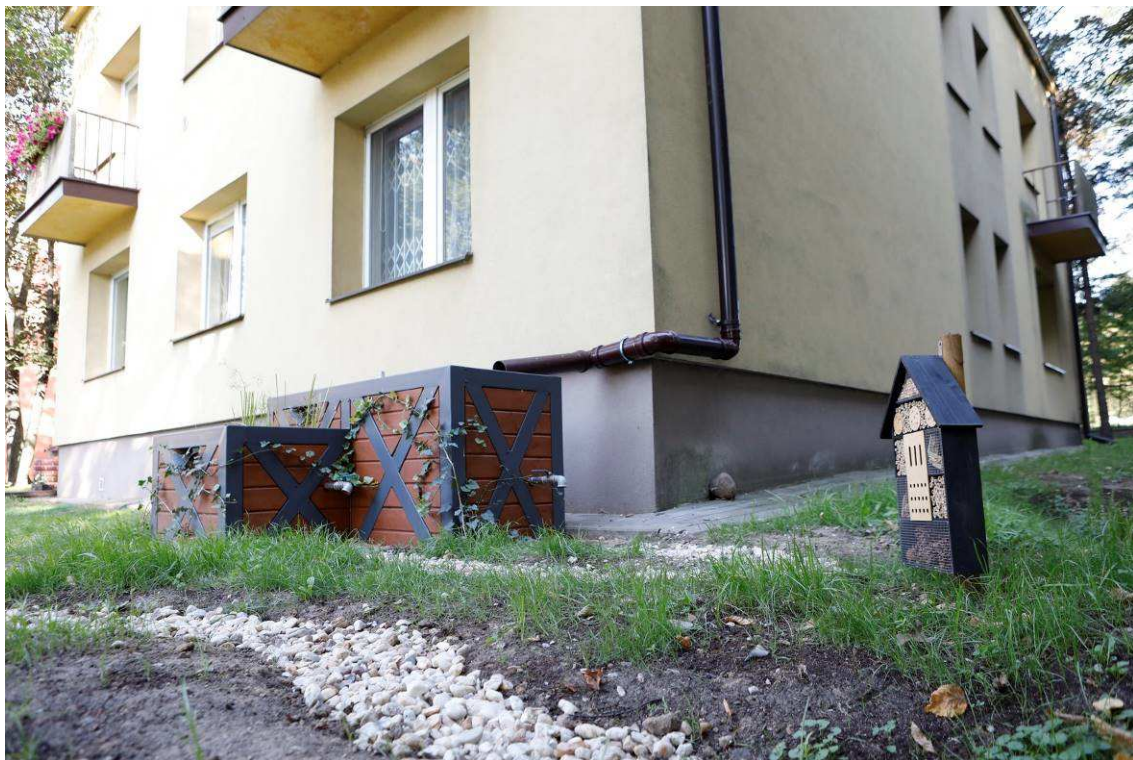
Picture 8 Appearance of the area after the construction- Swale - water supply by dry stream
