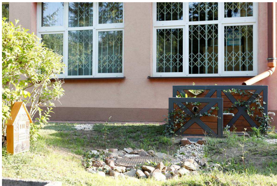
Picture 9 Appearance of the area after the construction- Climabox + Swale
