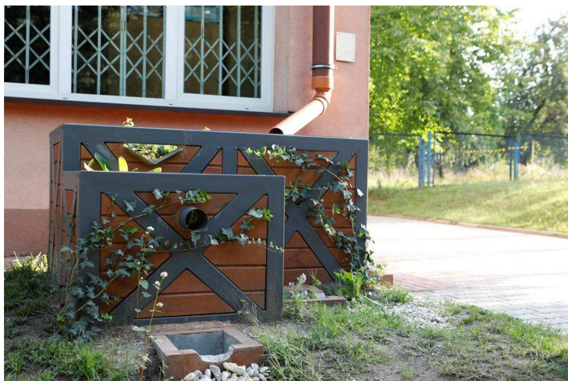
Picture 10 Appearance of the site after the construction- Climabox + Swale
