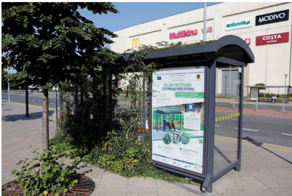
Picture 6 Appearance of the area after the construction- Tree trench
