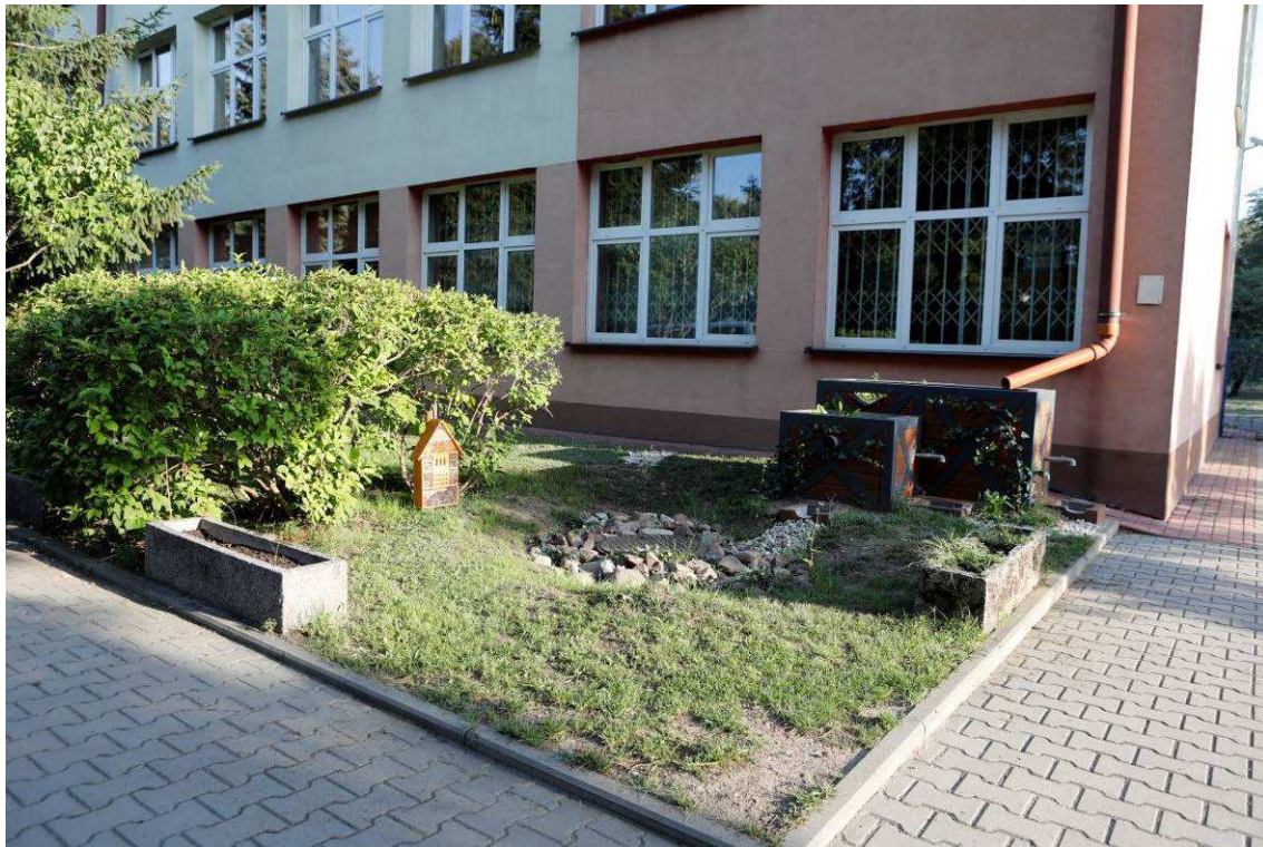
Picture 6 Appearance of the area after the construction- Climabox + Swale
