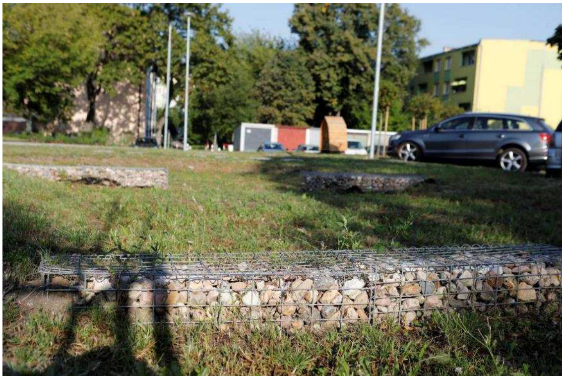
Picture6 Appearance of the site after the construction- Absorbent Swales - gabions
