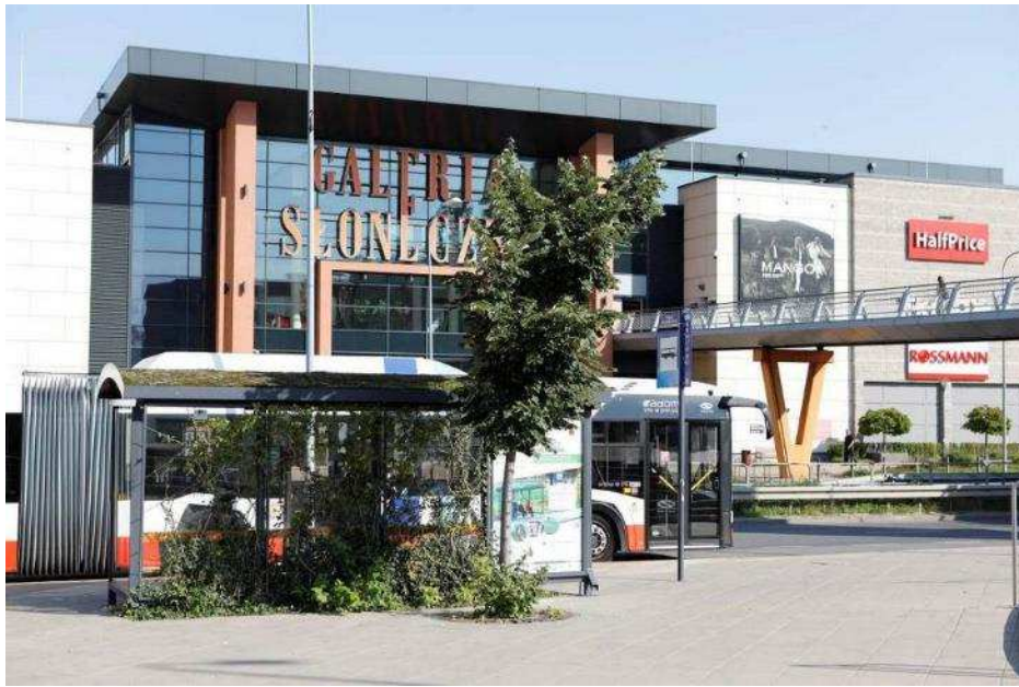
Picture32 Appearance of the area after the construction- Tree trench
