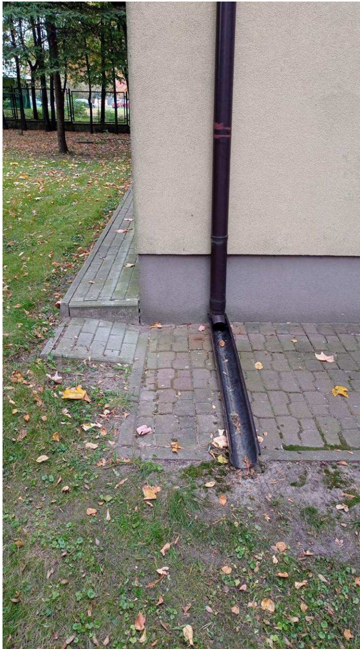
Picture41 area before the construction- Swale
