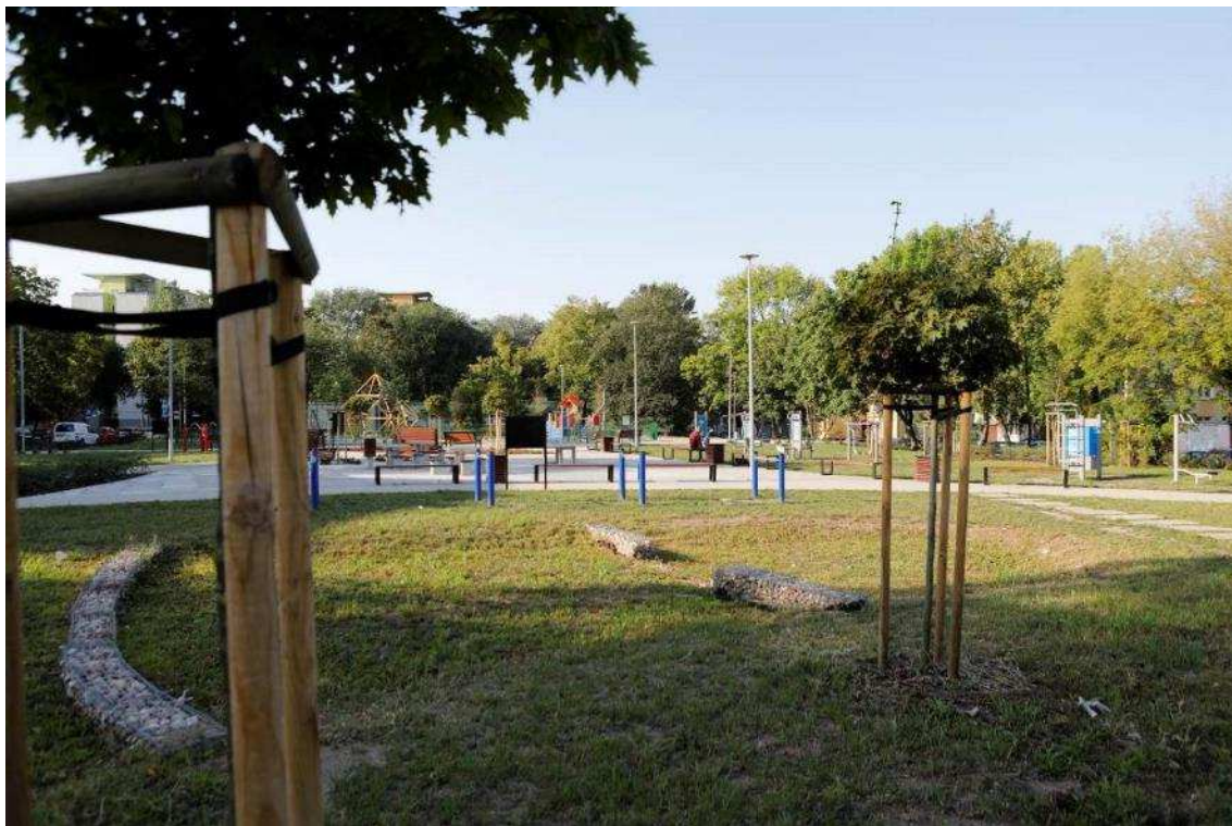
Picture8 Appearance of the site after Works Swales and tree plantings
