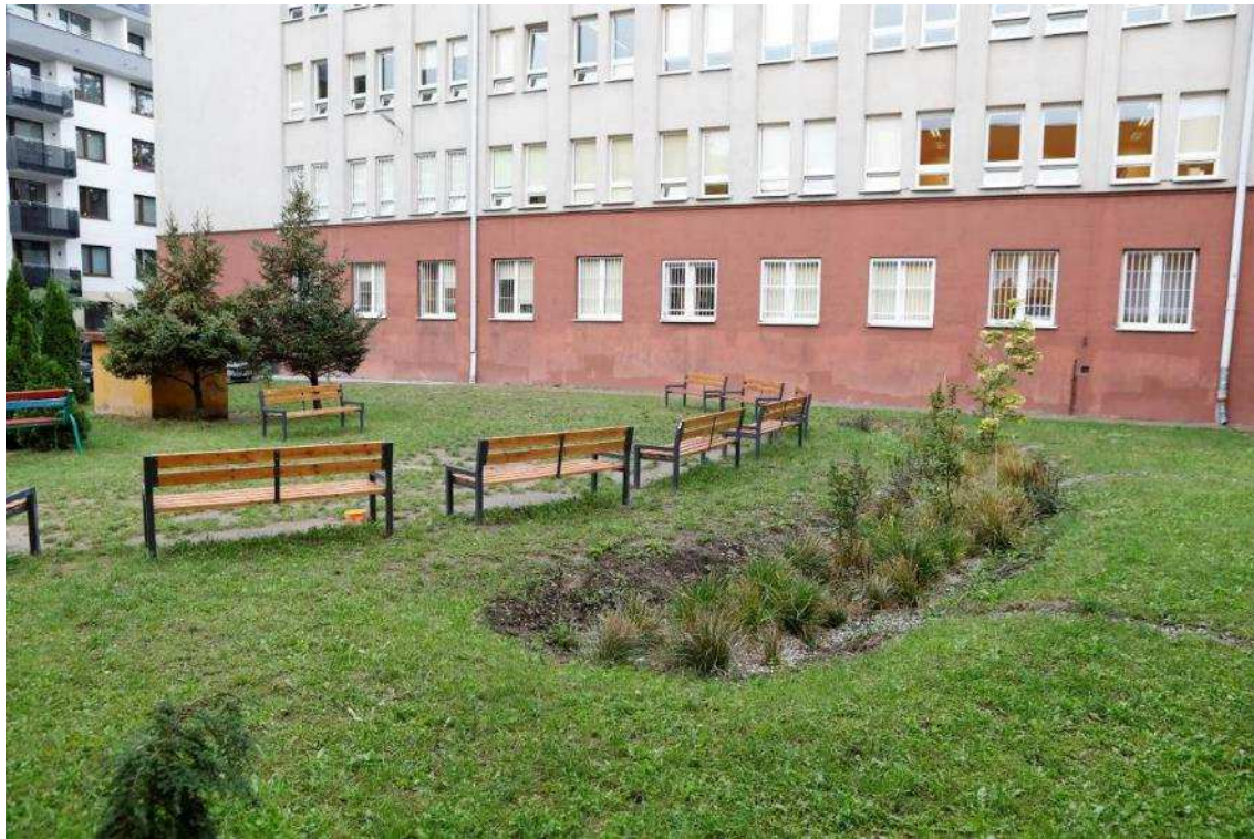
Picture 8 Appearance of the area after the construction- Swale with a row of trees + elements of small architecture
