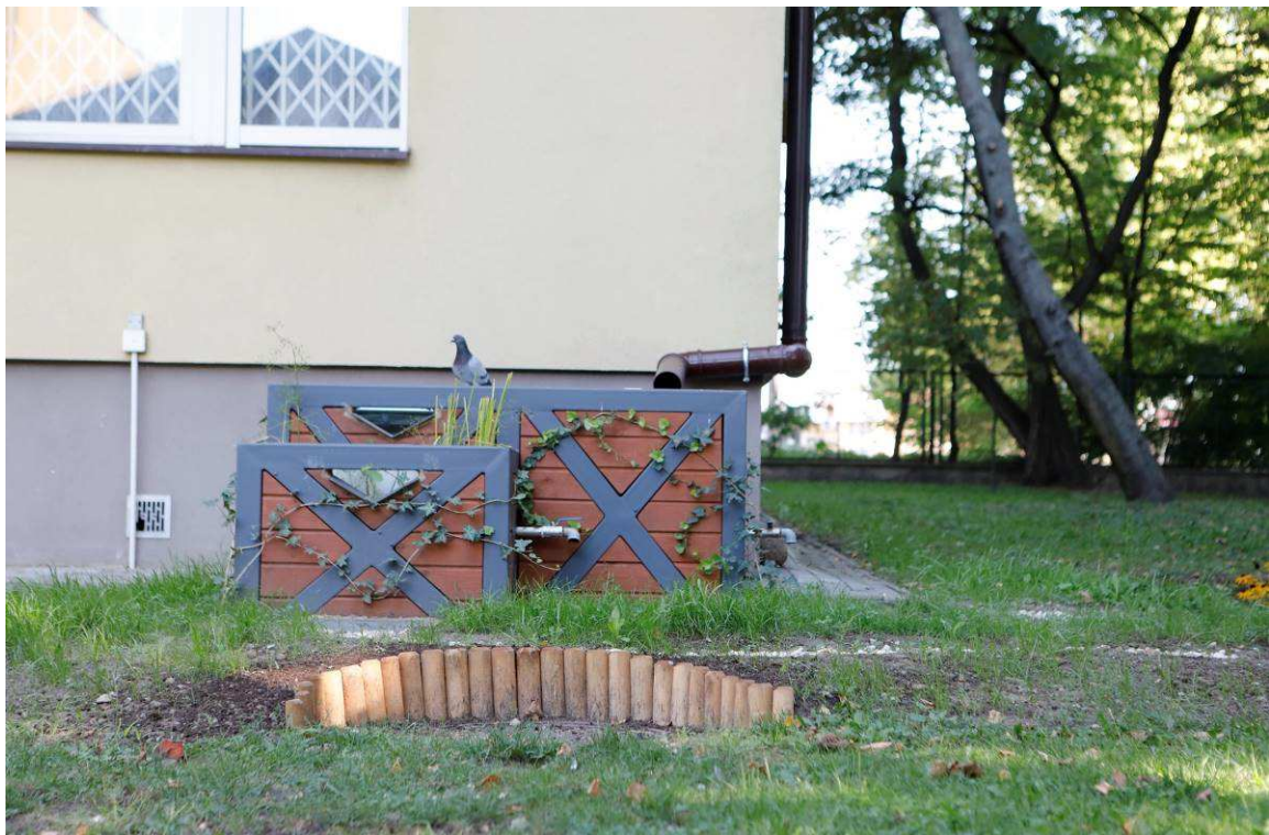
Picture 6 Appearance of the area after the construction- Swale
