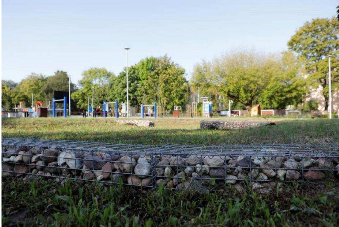
Picture7 site after the construction- Absorbent Swales - gabions
