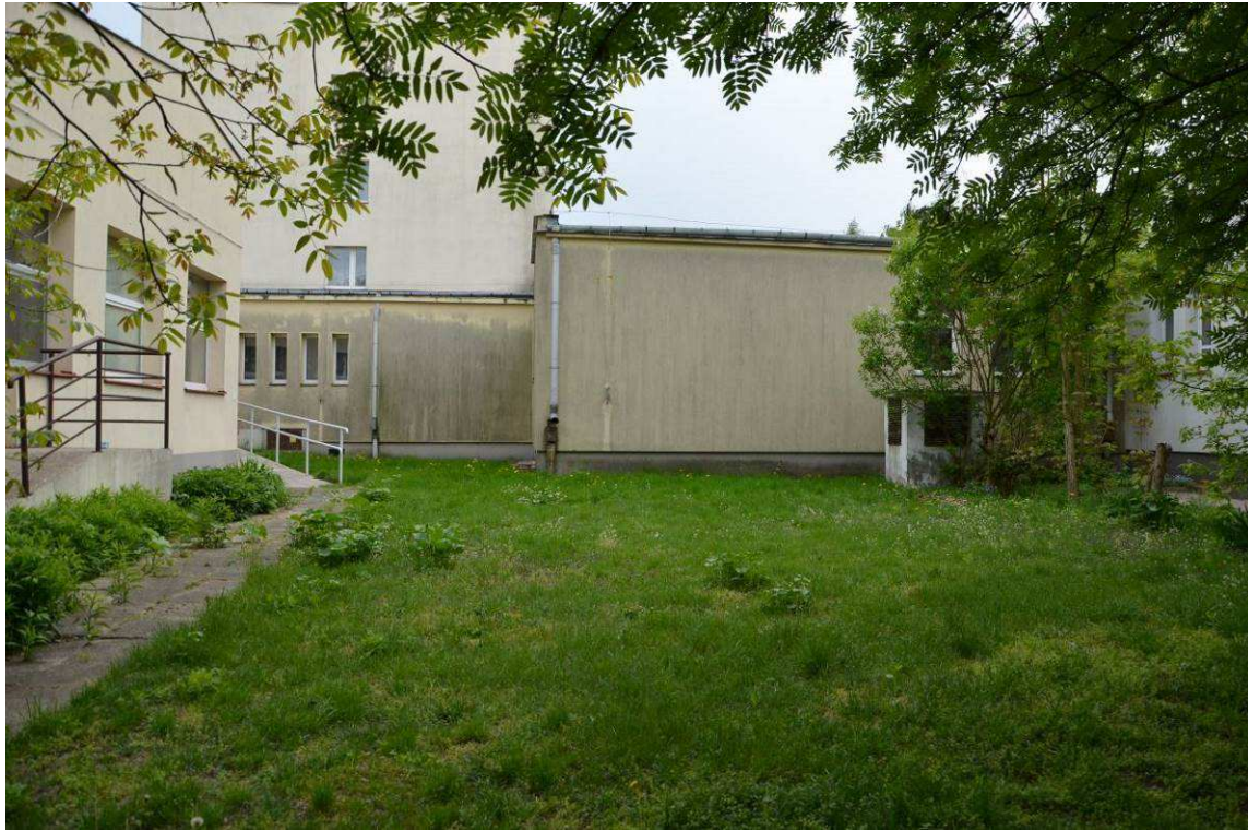
Picture36 area before the construction- Swale
