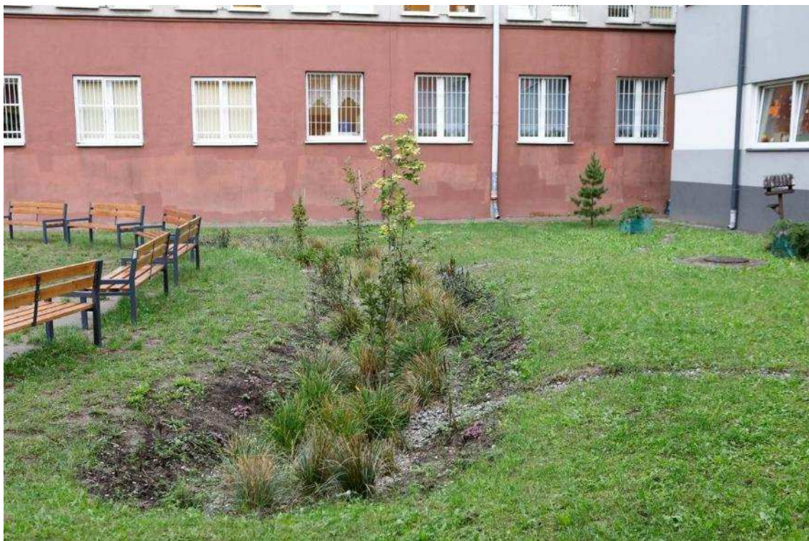
Picture 9 Appearance of the area after the construction- Swale with a row of trees + elements of small architecture
