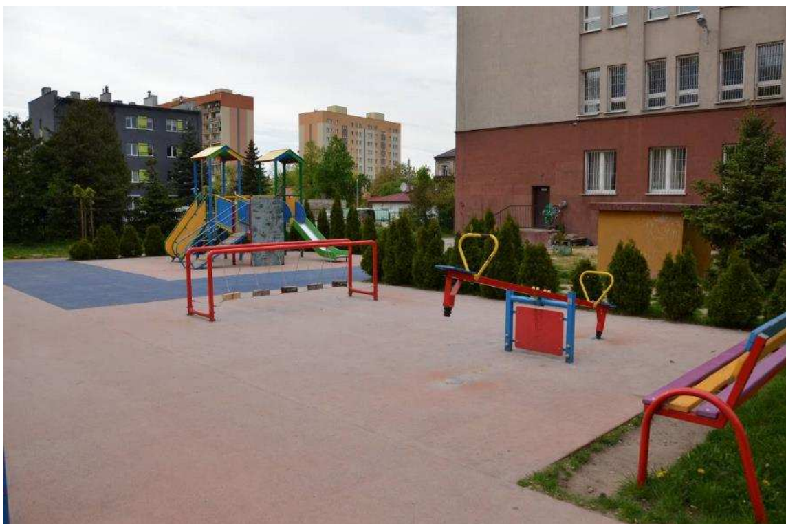
Picture31 area before the construction- Basins with a row of trees
