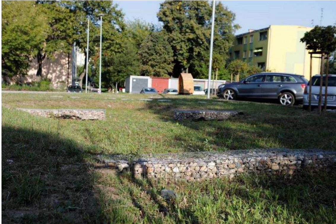
Picture5 Appearance of the site after the construction- Absorbent Swales - gabions
