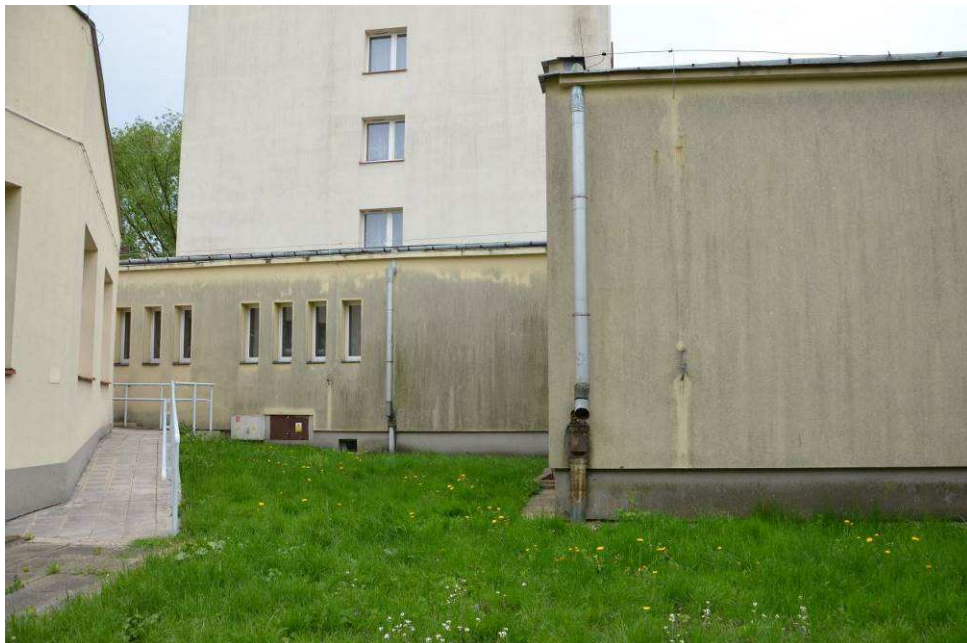
Picture37 area before the construction- Swale
