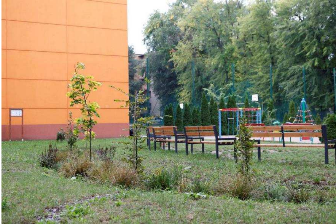
Picture 6 Appearance of the area after the construction- Swale with a row of trees + elements of small architecture
