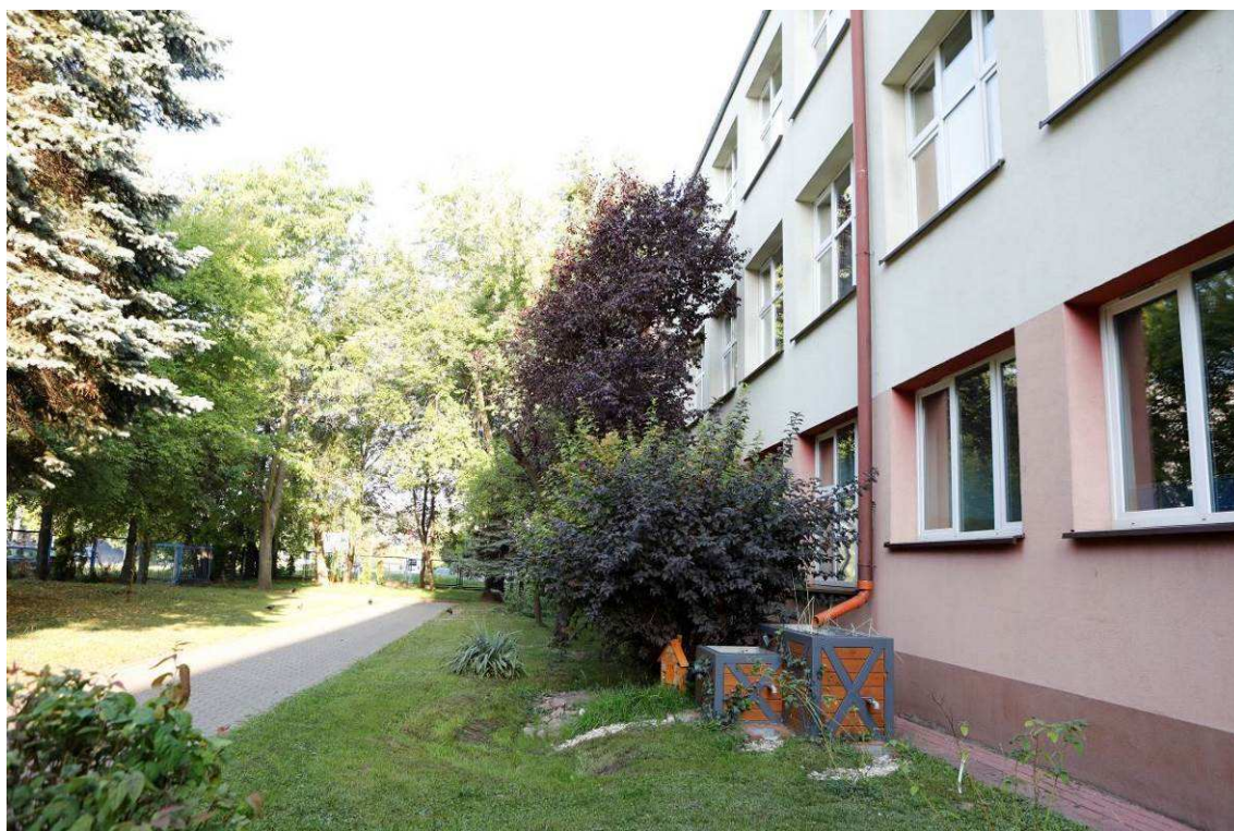
Picture 3 Appearance of the area after the construction- Climabox + Swale
