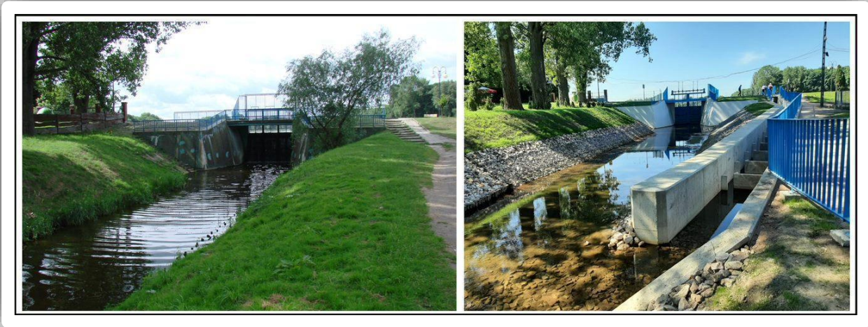
Photo 6. Main weir and fish pass on the Borki reservoir before and after the project. Own source
